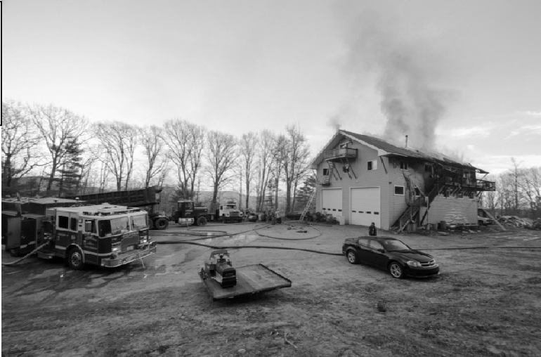
Gilford firefighters operate a building fire on Young Road – originally reported as Gilford – actually in Belmont. 4.17.13
