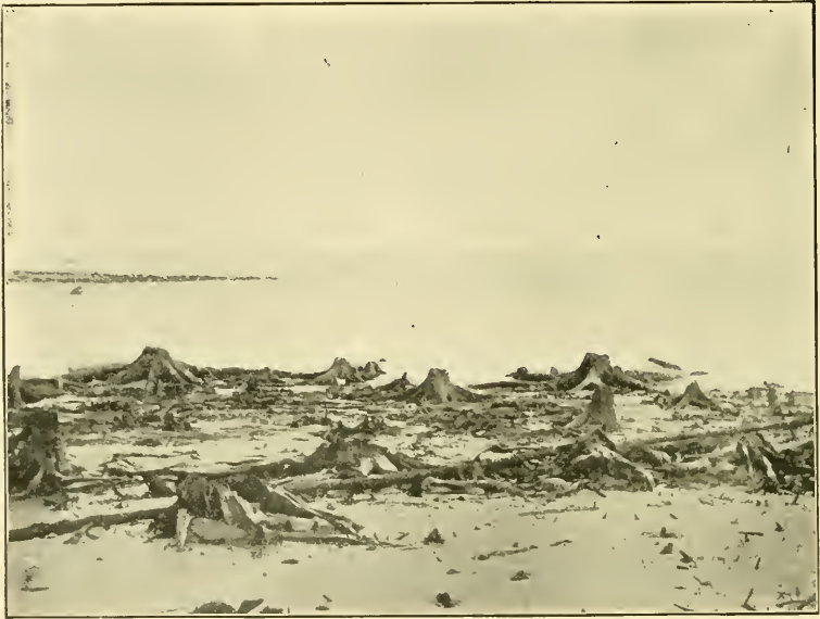
CEDAR STUMPS AND CABLE AT JENNESS BEACH.
