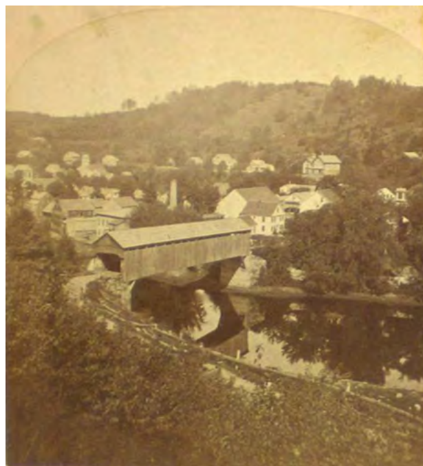
Depot Street Bridge
