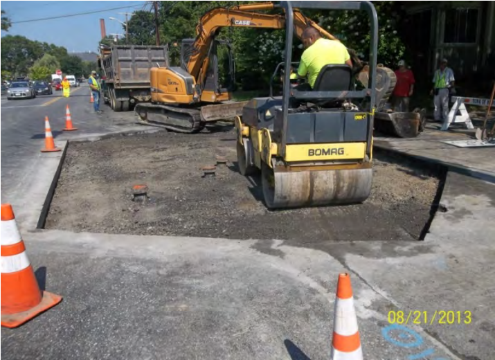
Preparing to pave at Summer Street
