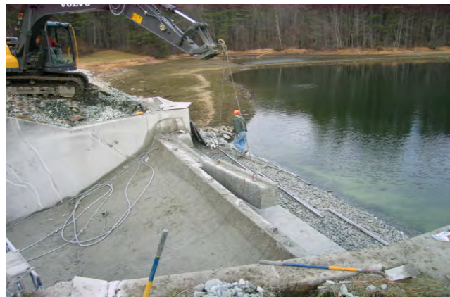
Removing Blocks from Spillway at Fletcher Reservoir
