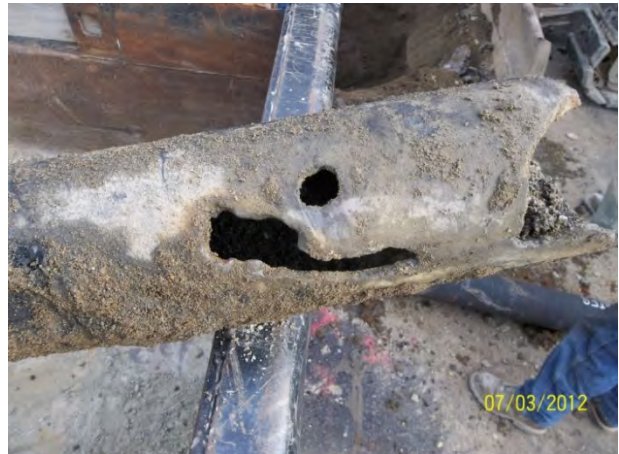
1893 Pipe from Lebanon Street
