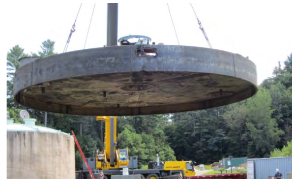
Old Digester Cover Removal
