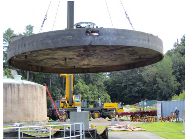
Old Digester Cover Removal
