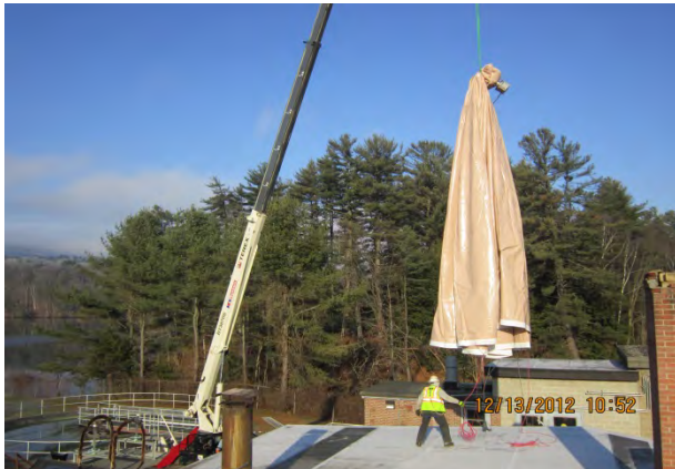
New Gas Holding Cover Installation
