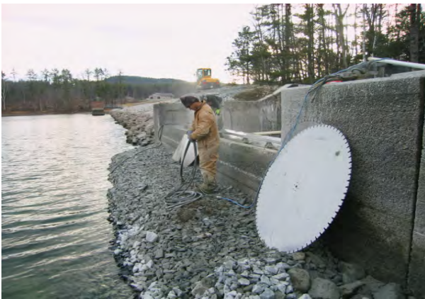
Cutting Spillway at Fletcher Reservoir
