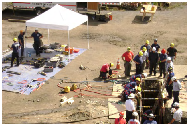
Members of the Hanover Fire Department participate in Trench Rescue Training
