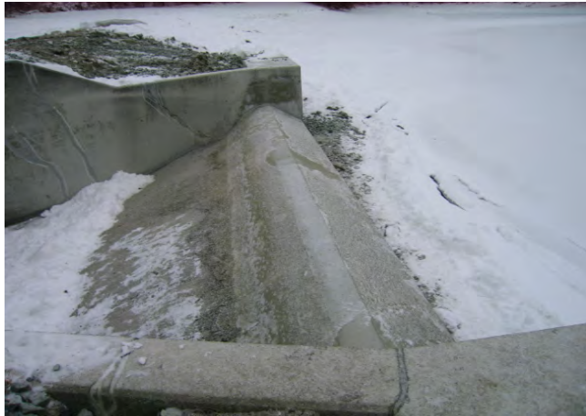
New Lowered Spillway Crest at Fletcher Reservoir
