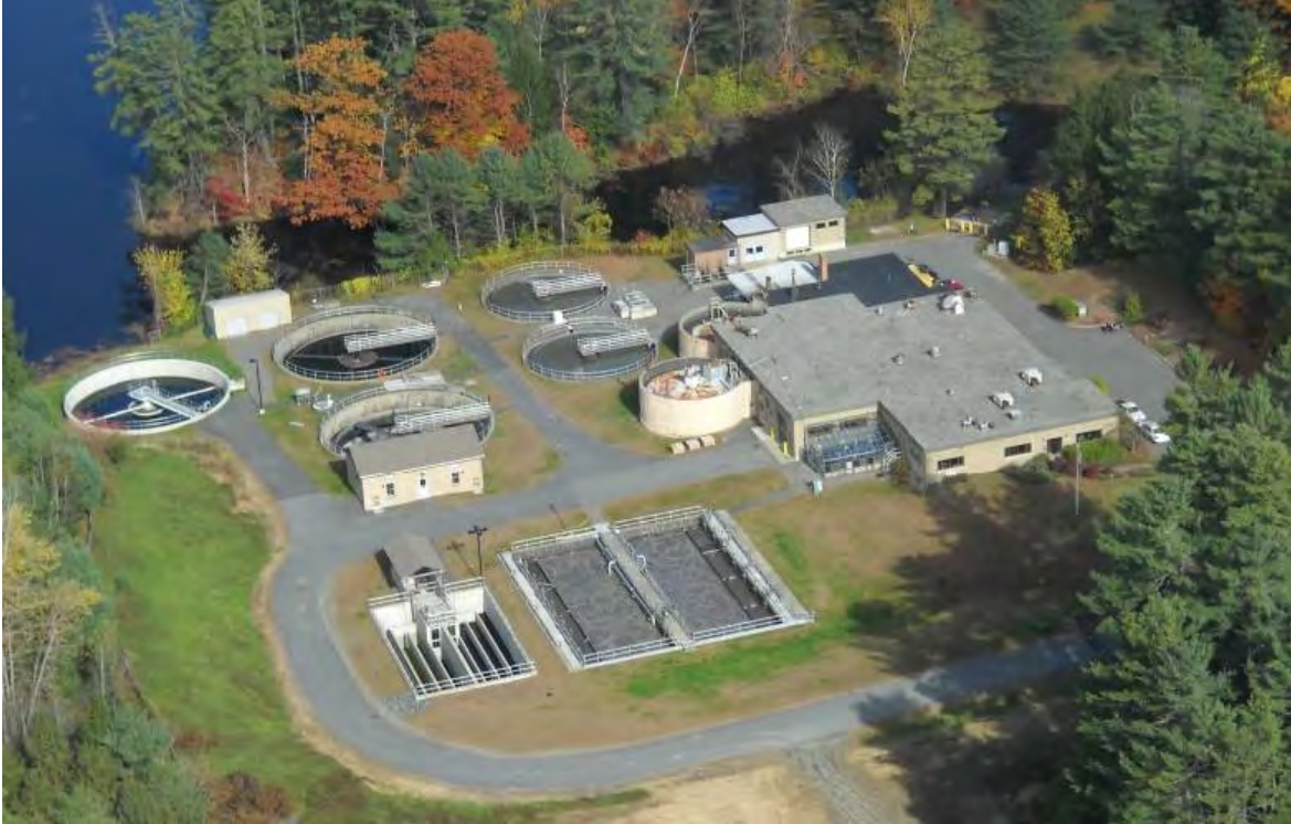
Facility aerial view
