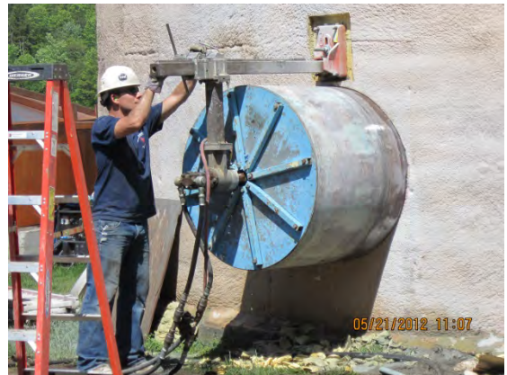
Digester Access Cutting
