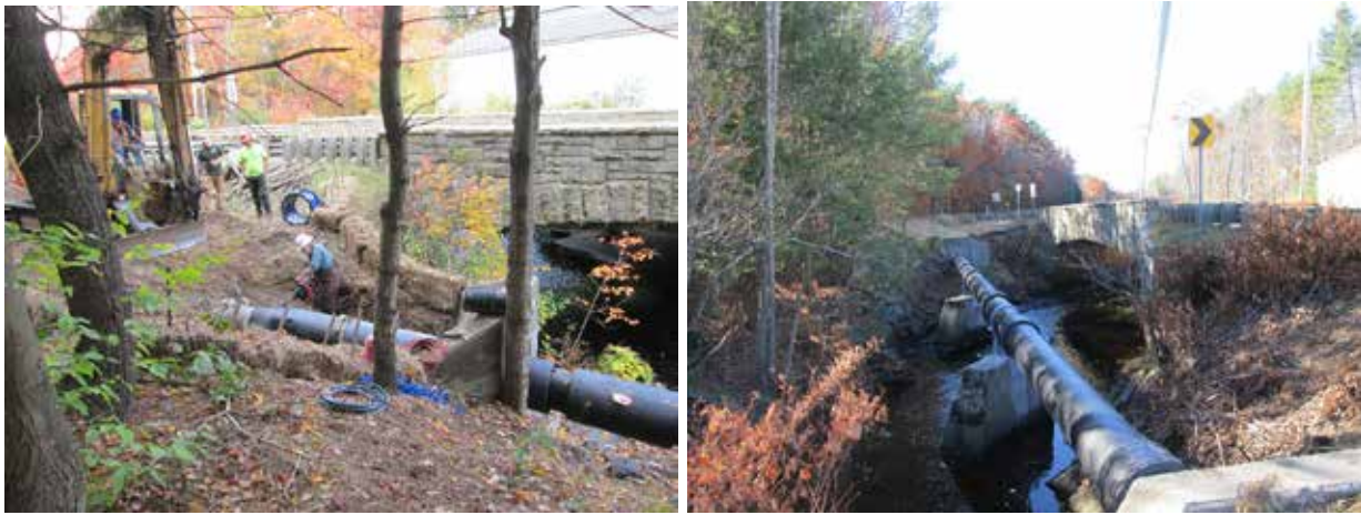
Sewer pipe bridge replacement project under construction and completed
