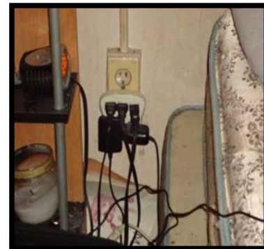
Unsafe Wiring
