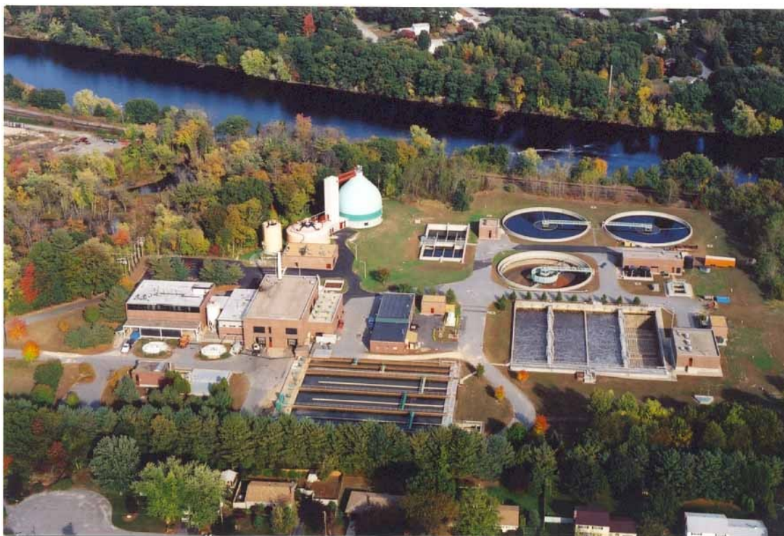
Wastewater Plant – 2008 Aerial View
