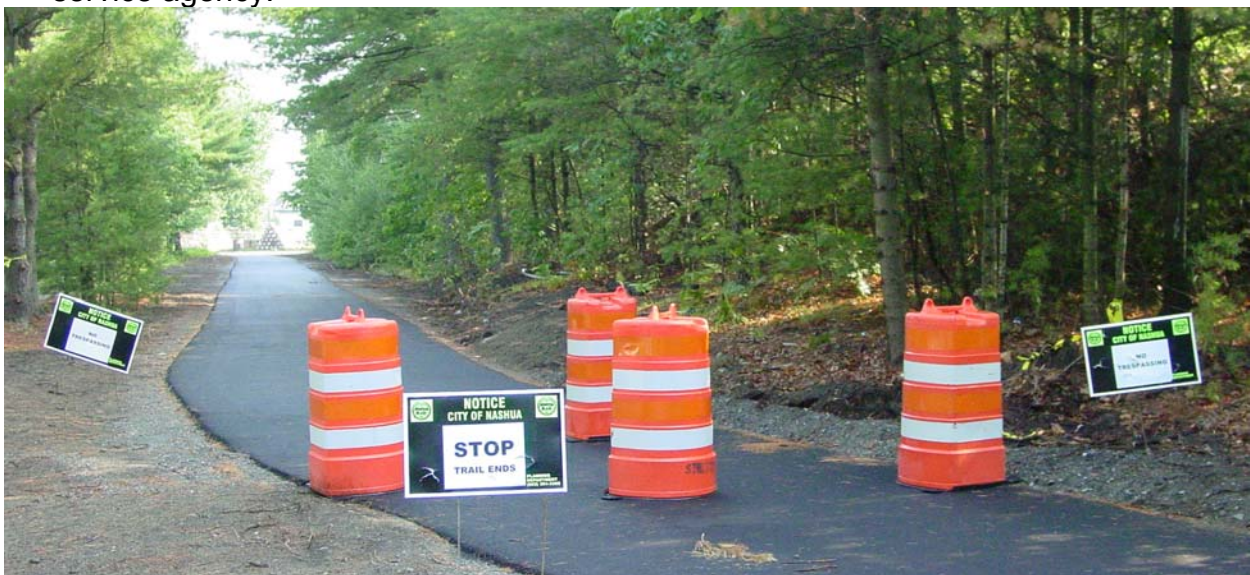
Paving of Nashua River Trail
