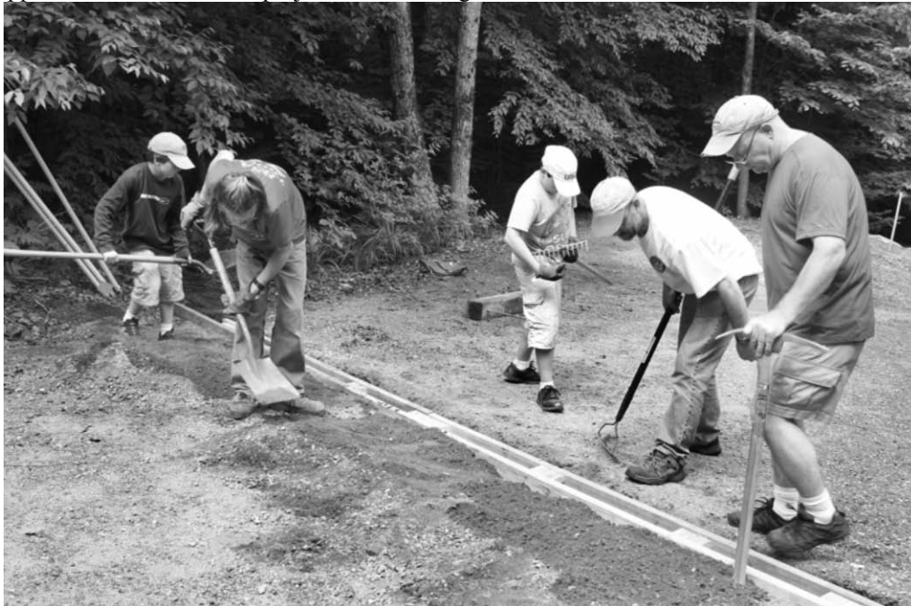
Again this year, Boy Scout Troop 71 & friends implemented Lake Conservation Corps stormwater management projects on Messer Pond properties. Shown here is an open box-top culvert.
