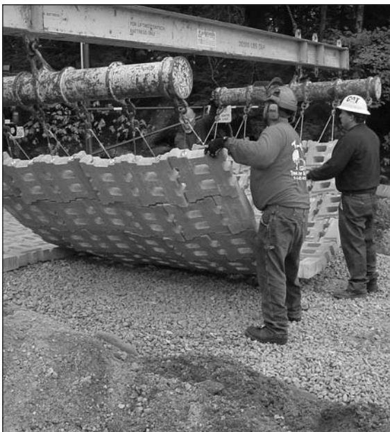
During the scheduled draw-down of Pleasant Lake, the boat launch was repaired using a mat made with fabric and stone, topped with blocks and then cabled together. By doing this work in-house, it saved the town about $35,000 and should help boaters get in and out of Pleasant Lake easier.
