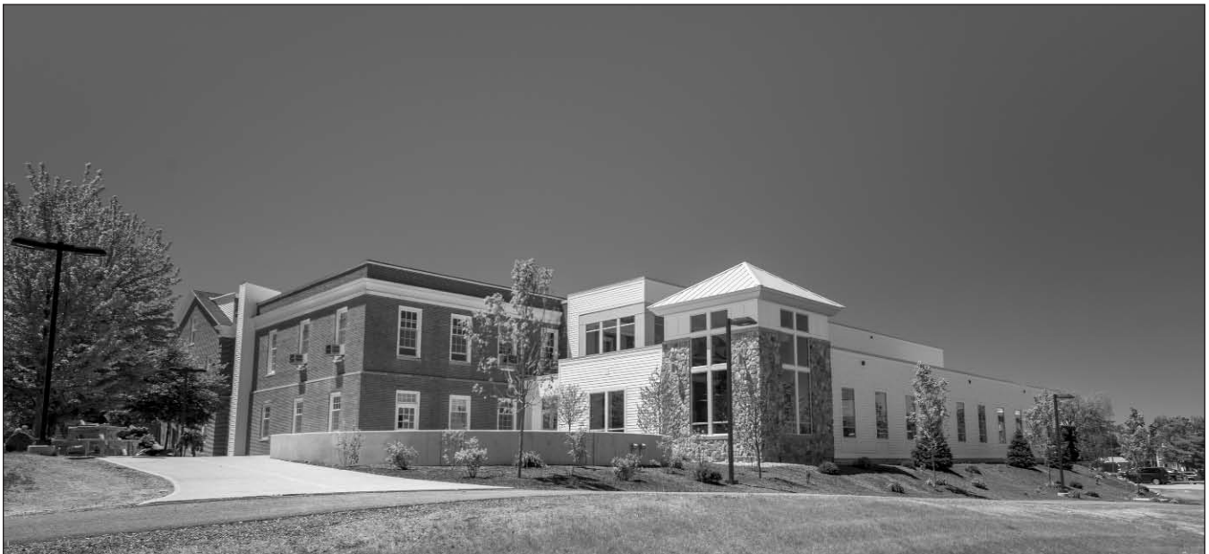
Addition to dining facility at Ware Student Center. Photo courtesy of Colby-Sawyer College
