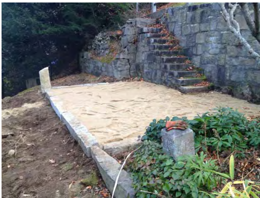
Boccelli patio under construction
