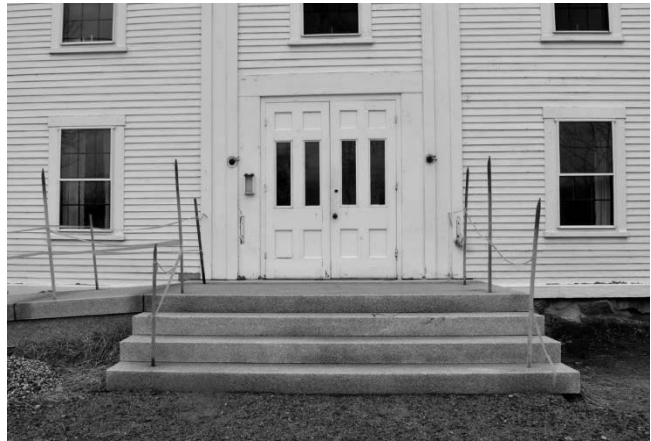
New steps at the Community Church
