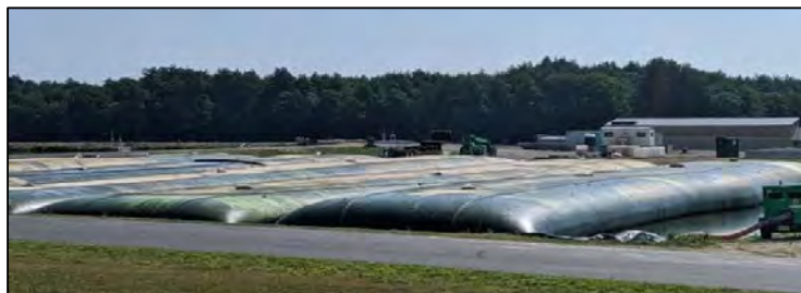
Geotubes dewatering wastewater biosolids on site. Photo by Matthew Berube.
