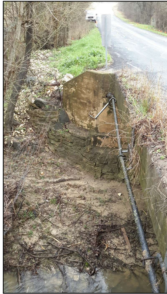
Figure 6. Boyce Lane bridge spanning Harris branch, eastern side of road facing south.
