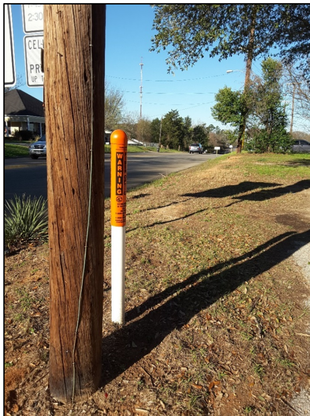
Figure 17. Raised telephone lines and buried fiber optic lines within the existing FM 16 ROW near Lindale, facing west.
