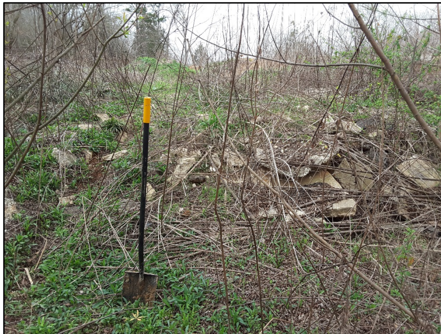
Figure 14. Large concrete boulders and asphalt push piles on southeastern edge of modified terrace of the mechanic's shop on parcel 50, facing west. Note the uneven terrace step (and riser) in the background depicting piles of added fill being pushed down the slope.
