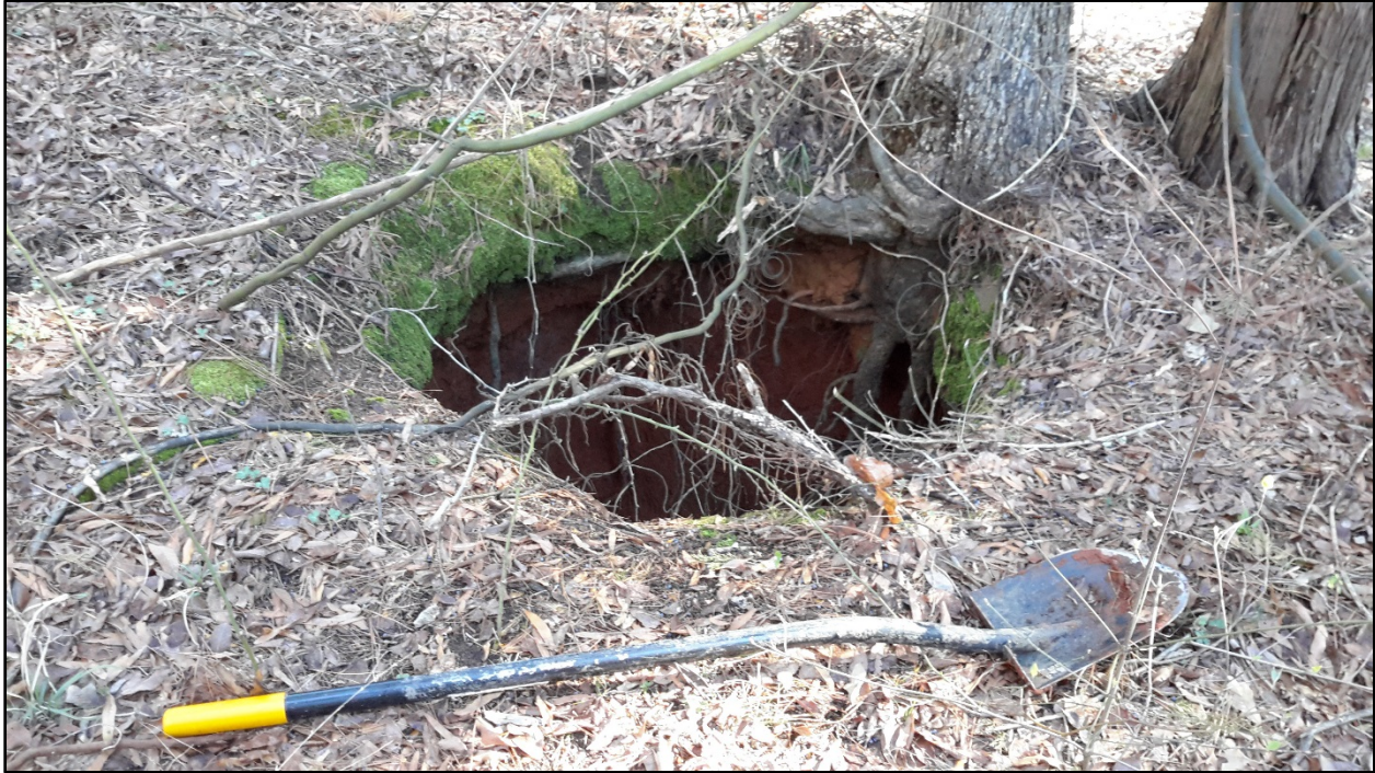
Figure 11. Sinkhole or eroded well located just outside the proposed ROW on parcel 12, facing northeast.
