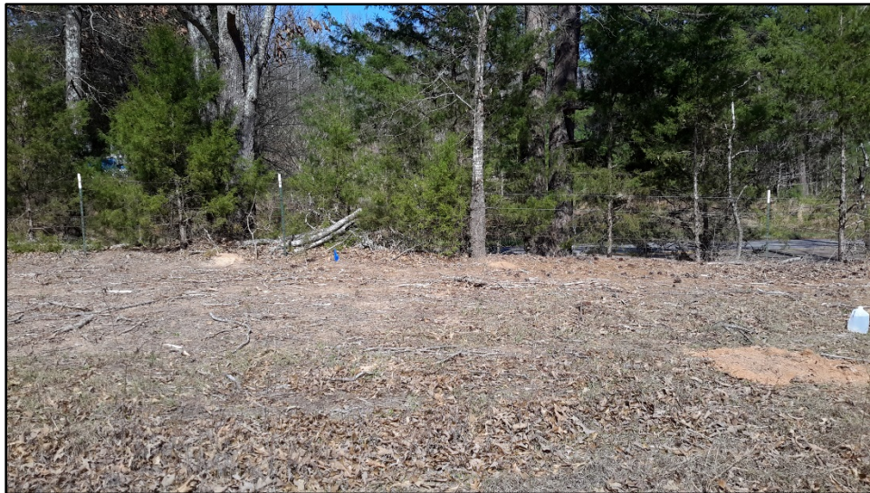
Figure 24. Site 41SM484 overview facing FM 16 with flagged buried water line in foreground, facing northeast on parcel 46.
