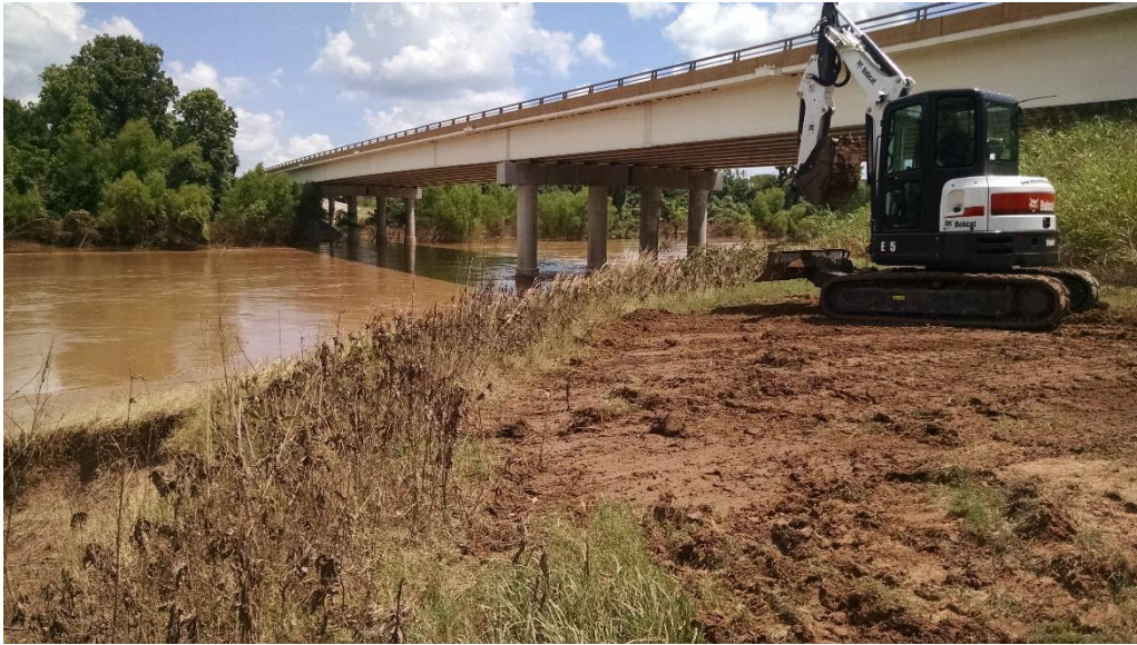
Figure 10. View of the general area surrounding backhoe trenches 1, 2, and 3.
