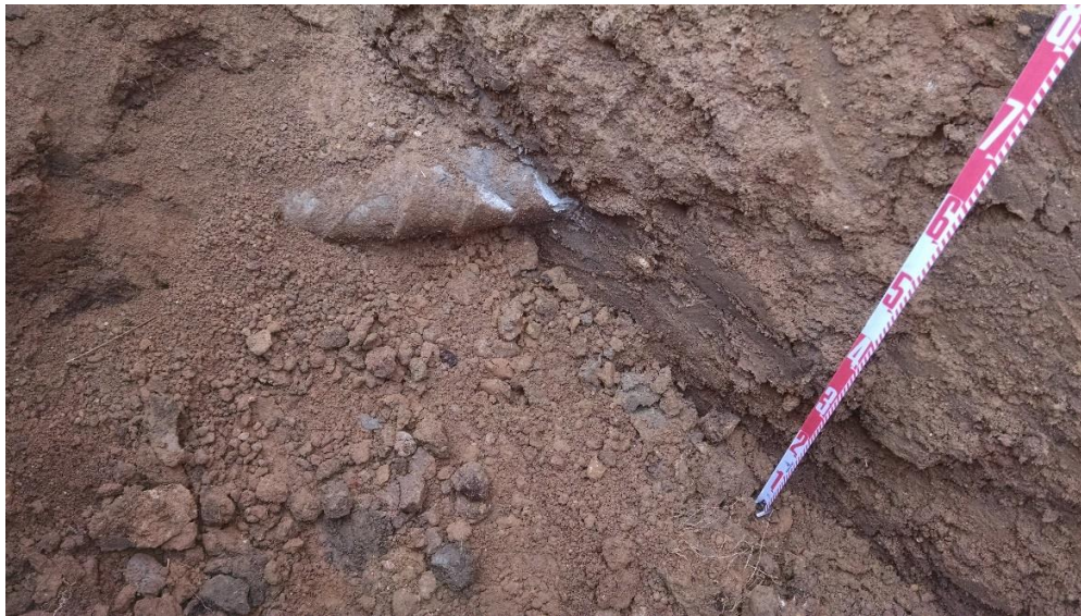
Figure 14. Detail of concrete spiral concrete stabilizing pillar in BHT1.
