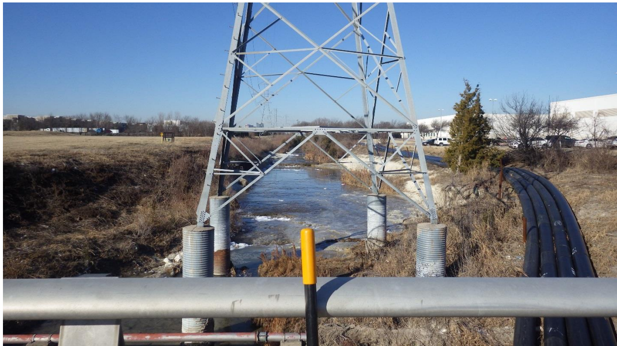
Figure 6. Overview of Beck Branch, showing utility disturbance. View facing to the west.
