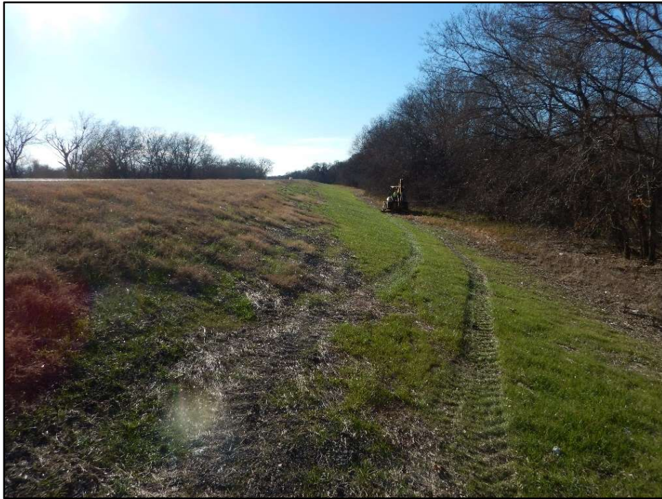
Figure 7. Overview of APE within existing ROW showing large fill section to elevate roadway above floodplain; fiber optic and other buried utilities along ROW margins precluded excavations in most of APE, facing southwest.
