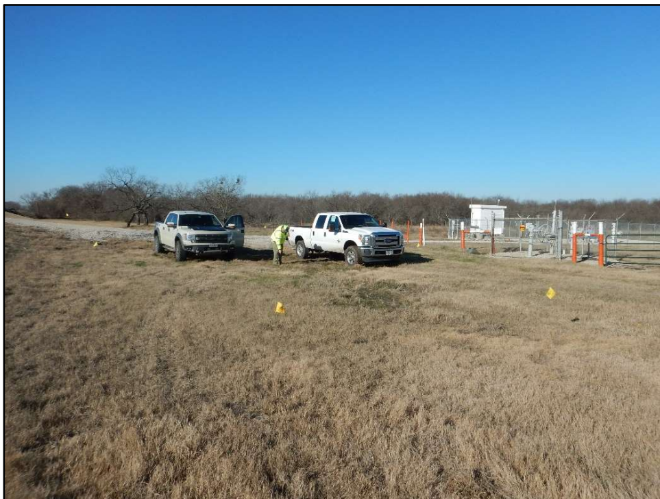
Figure 8. Overview of APE showing common disturbances within the APE; including multiple parallel buried utilities, pipelines, driveways, and road fill, facing southeast.
