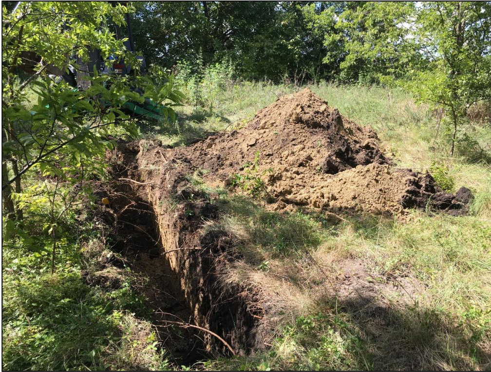
Photo 7. View of Backhoe Trench 1. View to the north.
