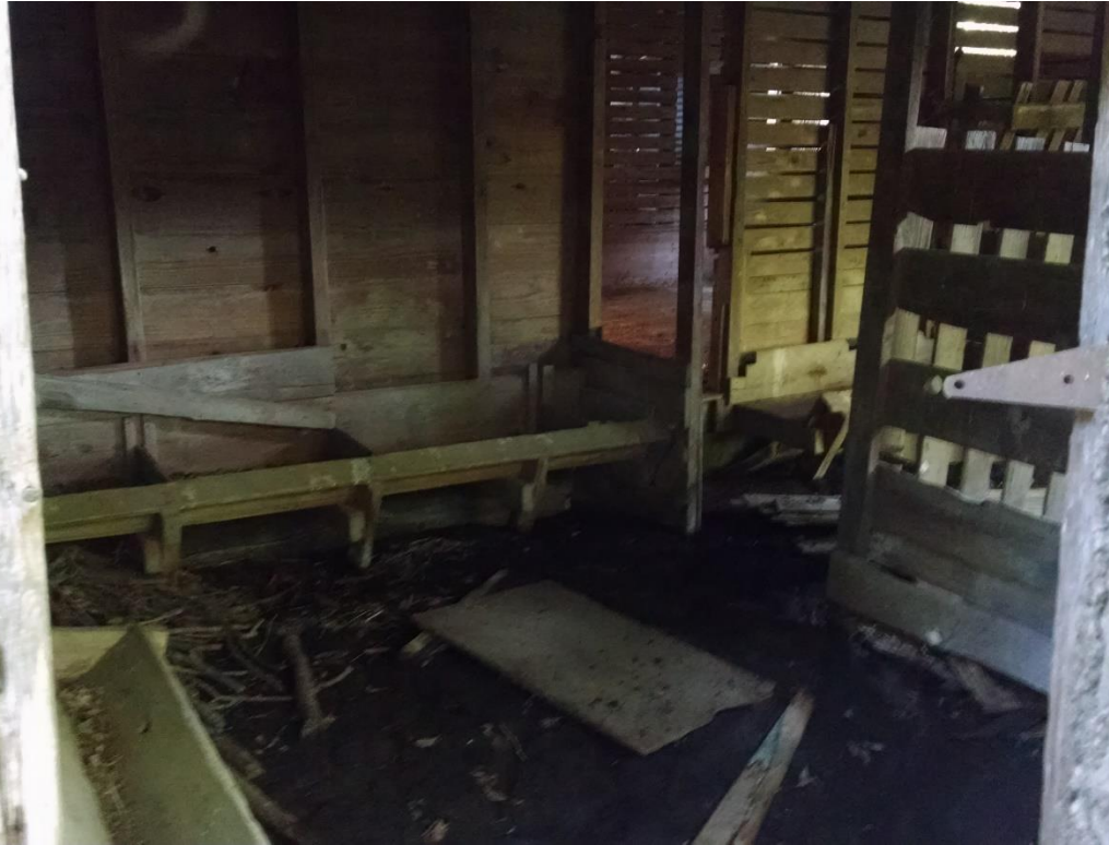
Photo 15. Interior of Outbuilding #1 at 41COL301.
