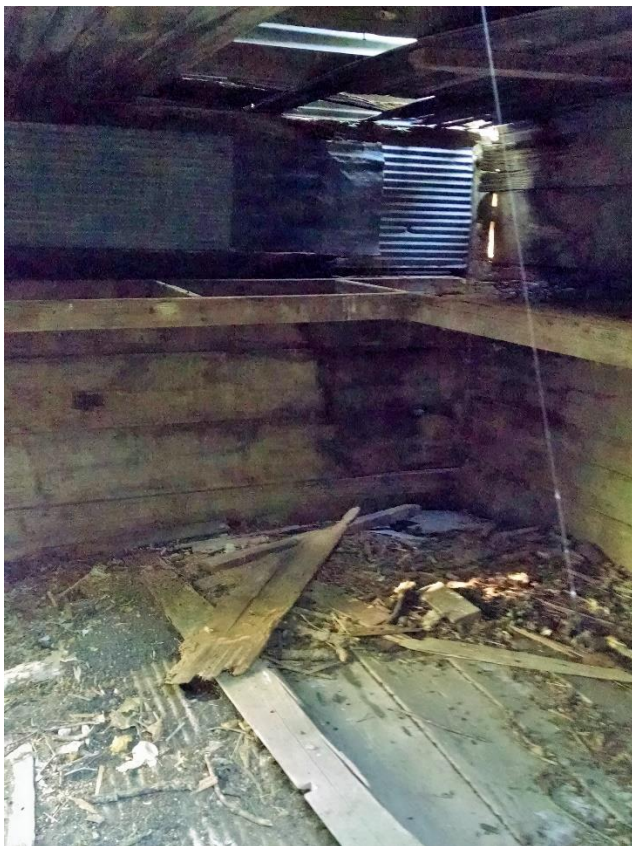
Photo 20. Interior of Outbuilding #4 at 41COL301.
