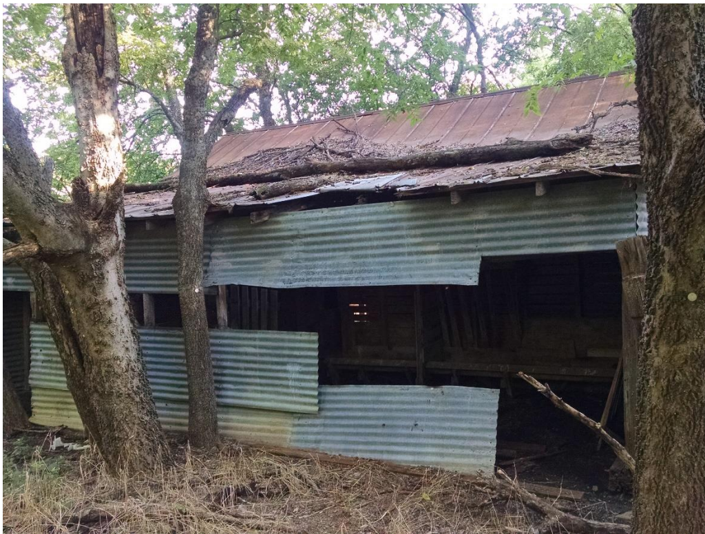
Photo 14. View of Outbuilding #1 at 41COL301. View to the northwest.
