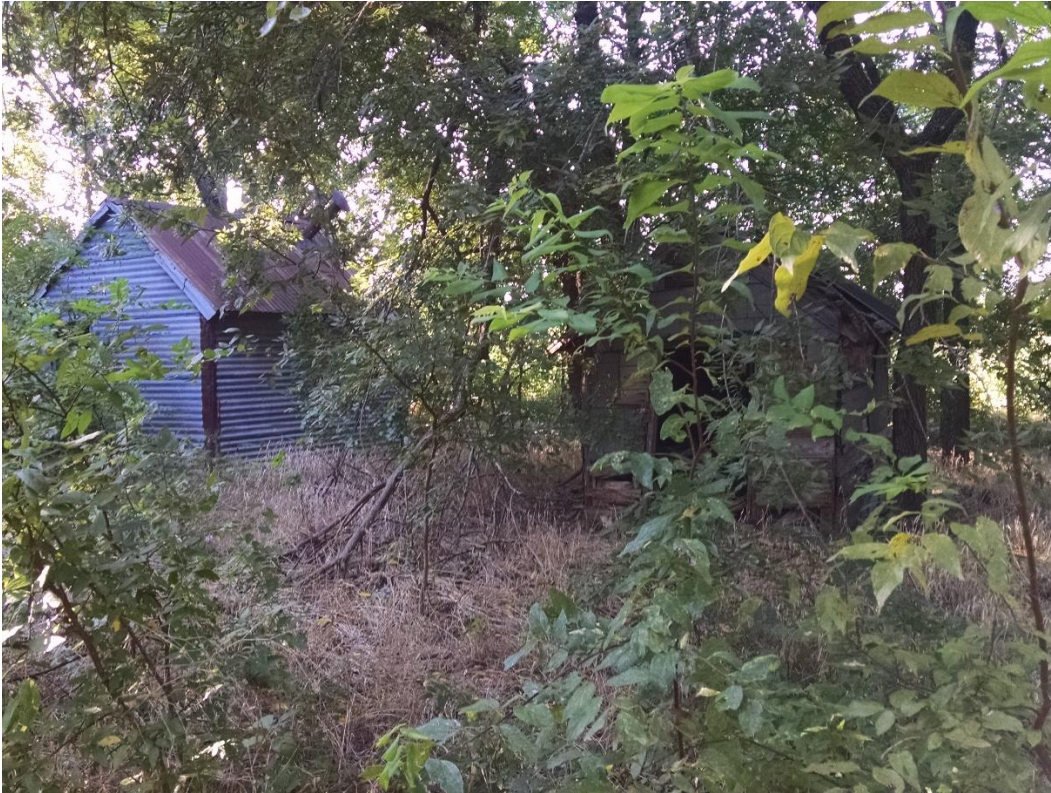
Photo 17. Outbuildings #3 and #4 at 41COL301. View to the southeast.
