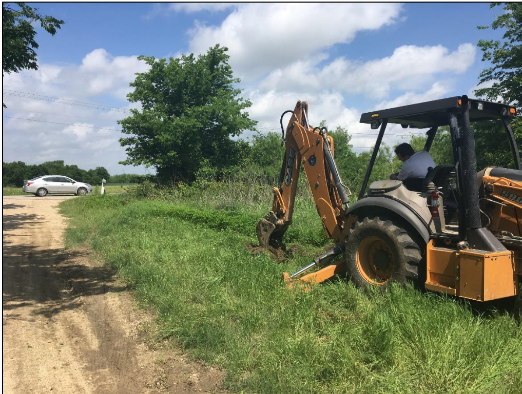
Photo 7. Excavation of Backhoe Trench 1. View to the west.
