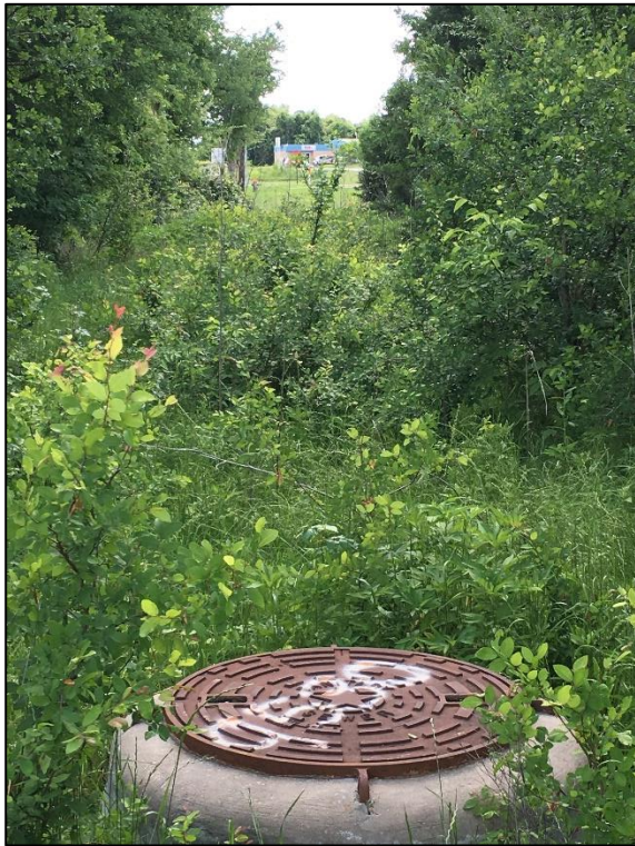
Photo 1. Southern end of alignment. Note sewer line. Other utilities in background. View to the south.
