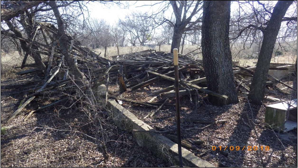
Figure 13. Collapsed barn outside the survey corridor. View is to the southeast.
