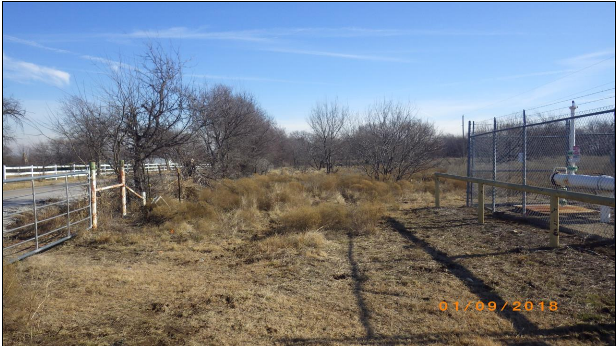
Figure 12. Looking down the centerline towards ST7 near the Atmos Facility. View is to the northeast.
