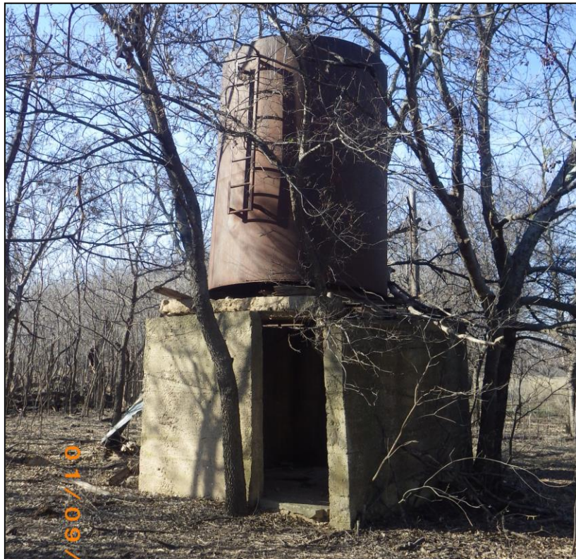
Figure 14. Structure with tank outside the survey corridor. View is to the southwest.
