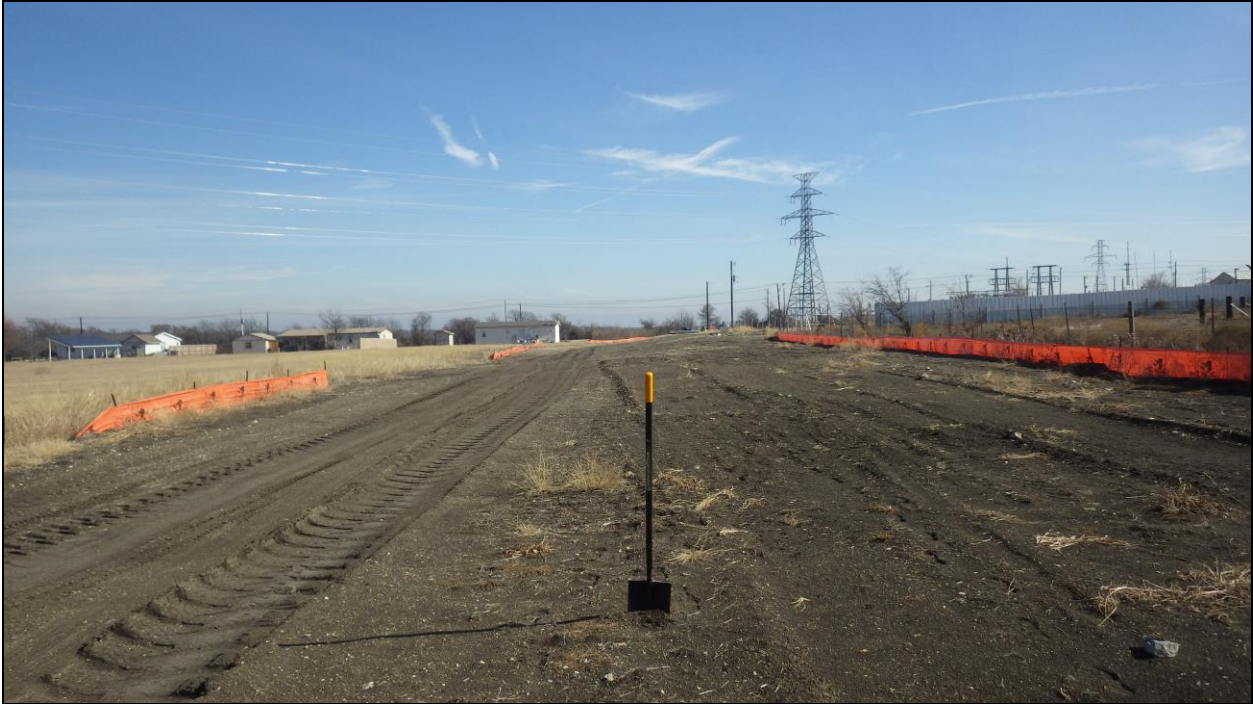
Figure 9. Construction disturbance within survey route, ST26-27 were not excavated. View is facing east.
