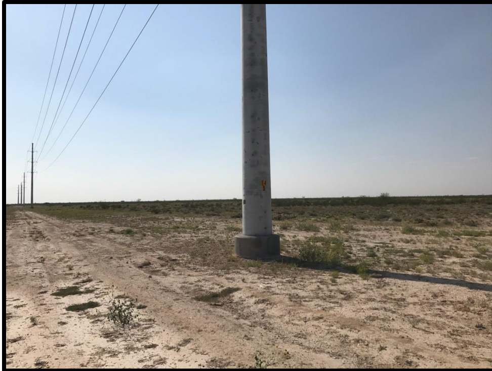
Figure 83. Overview of Monopole Structure 14/5, on University Lands, Facing Northwest
