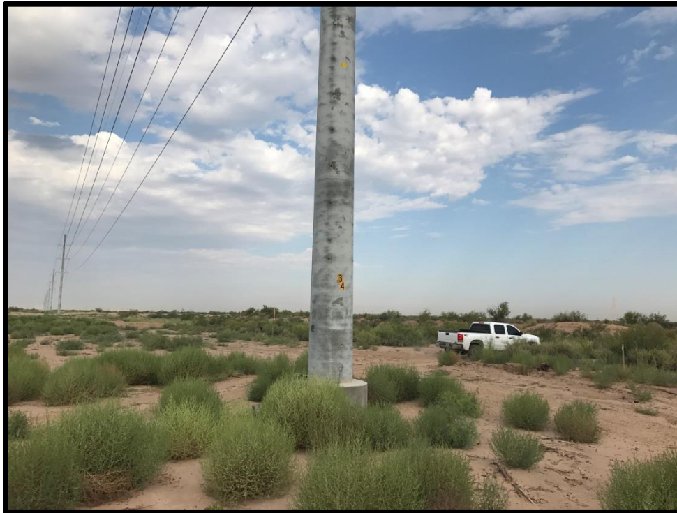
Figure 87. Overview of 41RV128, Facing West
