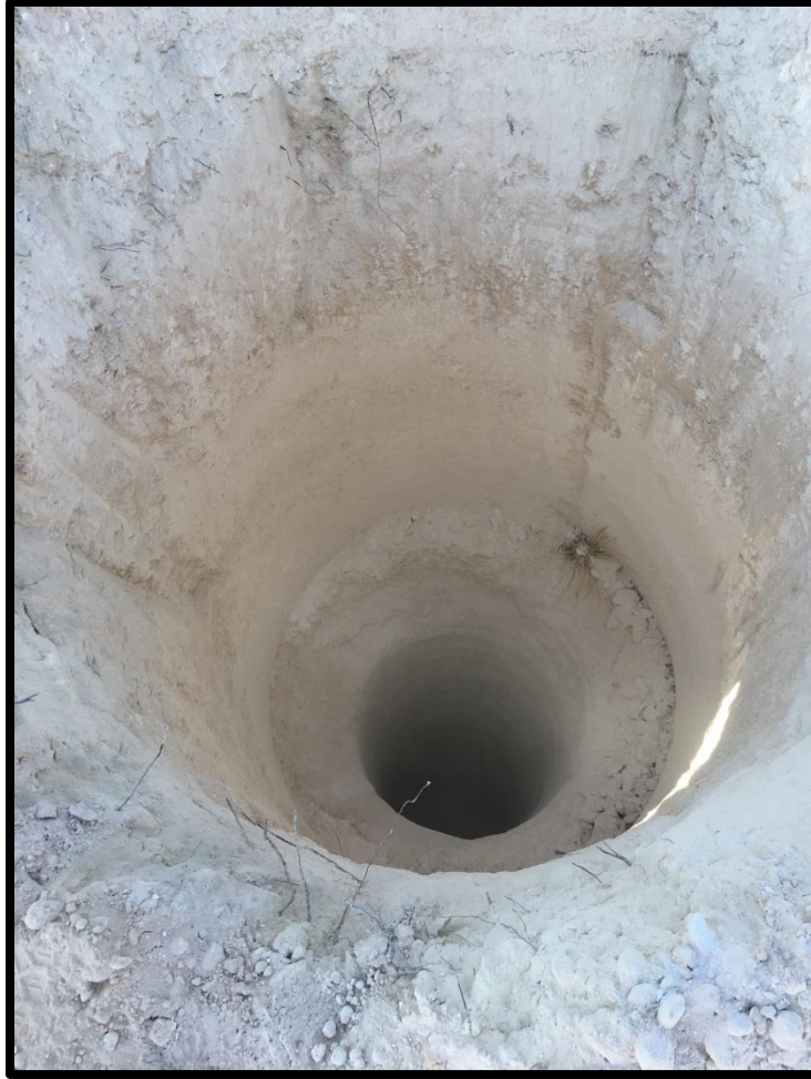
Figure 80. Completed Auger Hole at Structure No. 56/3 at Site 41CU835
