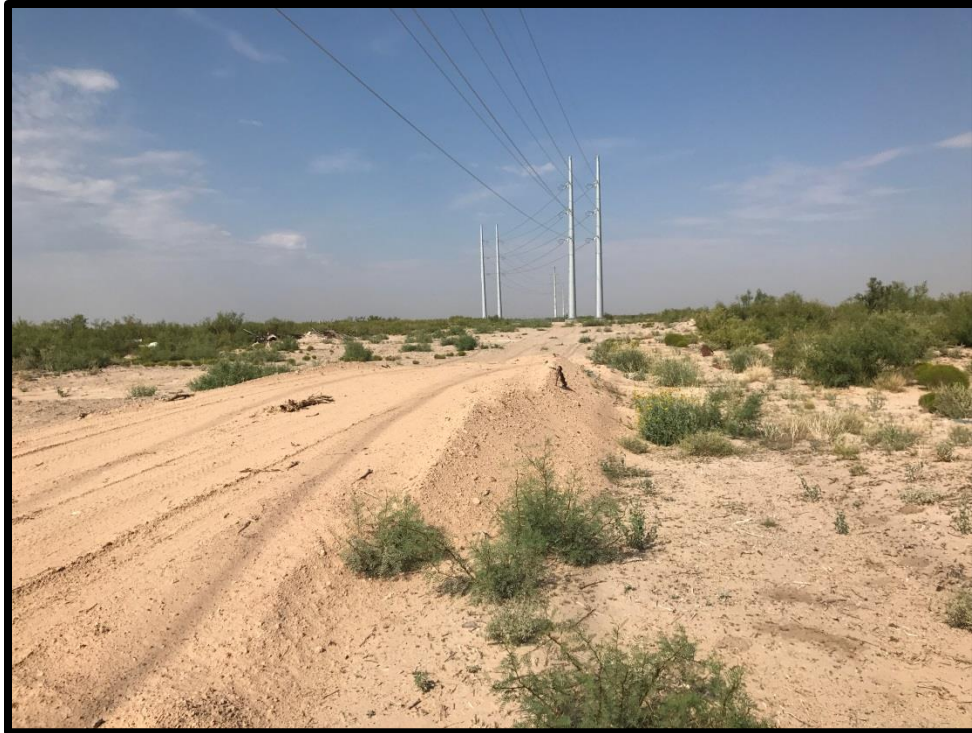
Figure 90. Overview of 41RV129, Facing West
