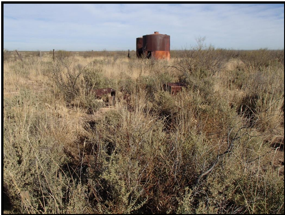
Figure 46. Overview of Silos Near 41WR97, Facing North
