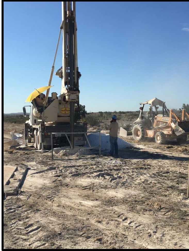
Figure 79. Auguring at Structure No. 56/3, at Site 41CU835, Facing Southeast
