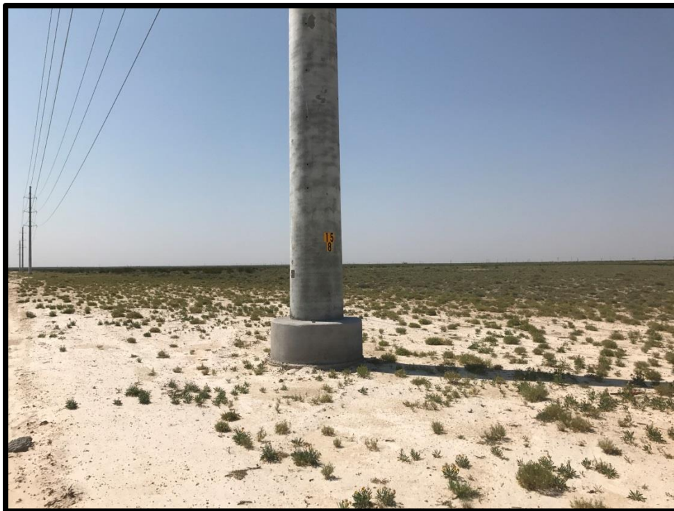
Figure 82. Overview of Monopole Structure No. 15/8, on University Lands, Facing Northwest
