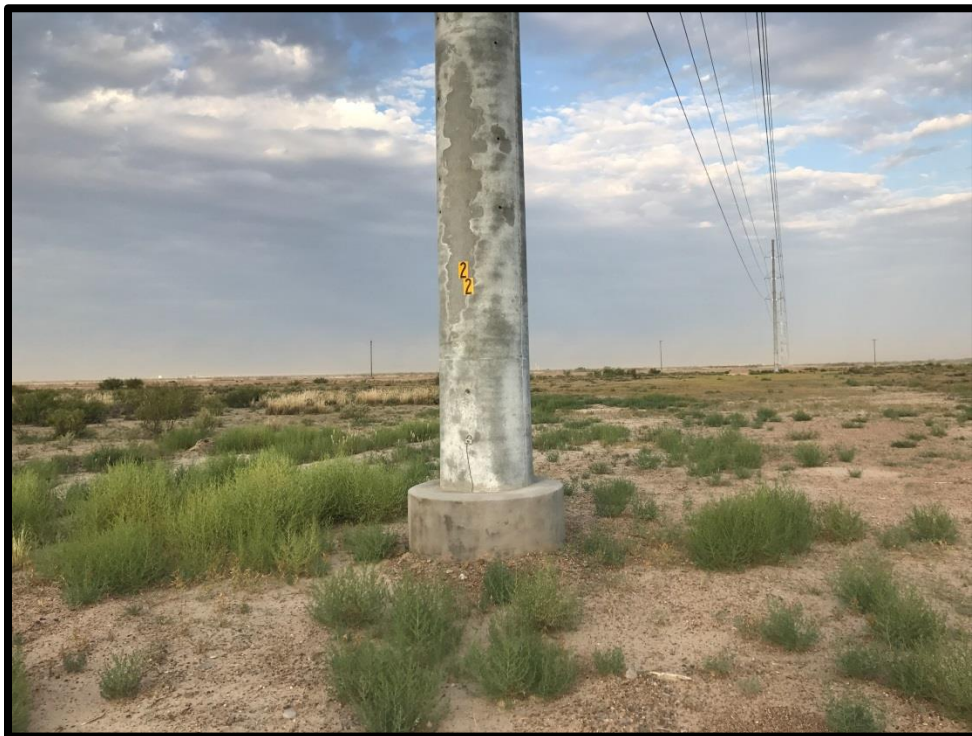
Figure 84. Overview of Monopole Structure No. 2/2, on the Eastern Pecos River Floodplain, Facing West
