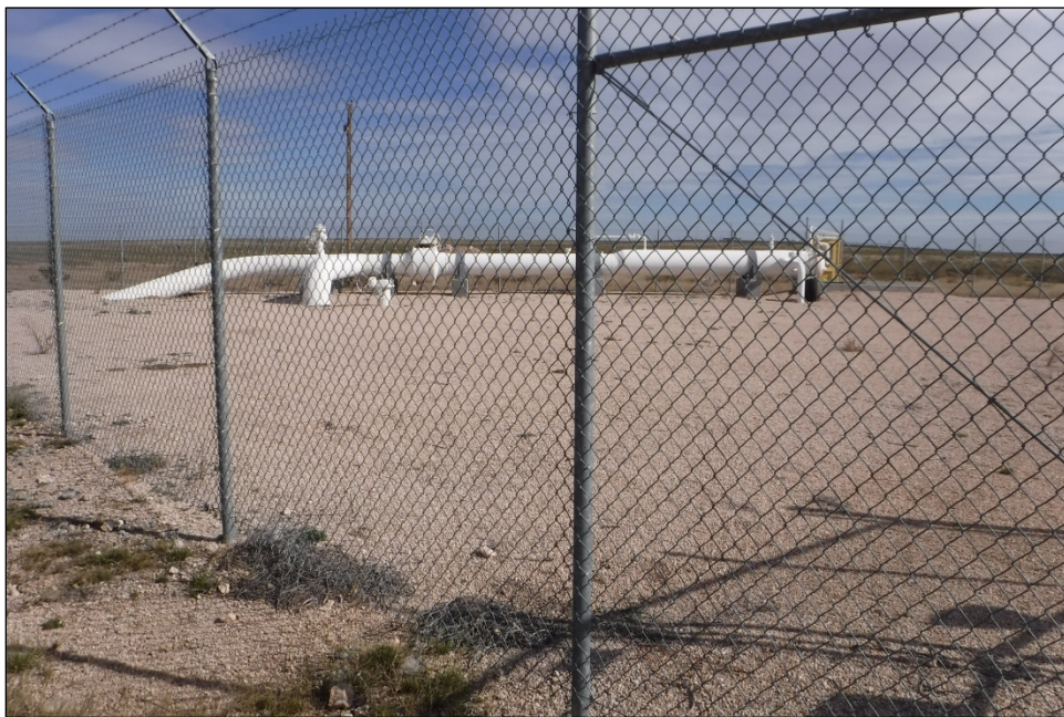
Figure 2.2 Station No. 142, existing pig trap overview looking east
