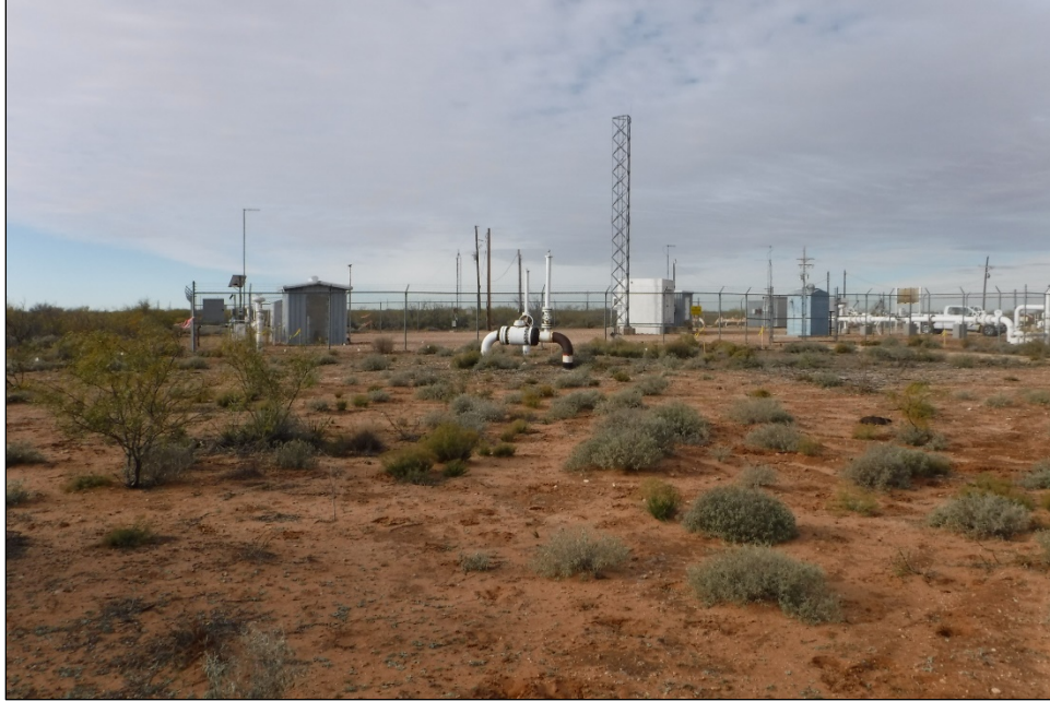
Figure 2.5 Oasis Meter Station looking east
