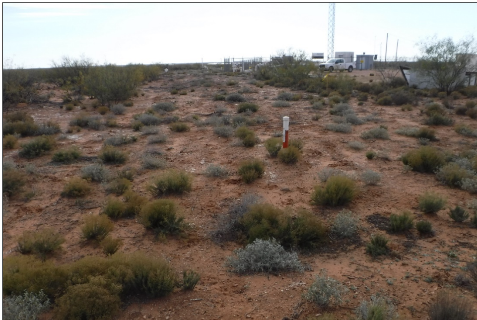
Figure 2.6 Oasis Meter Station pipeline looking east
