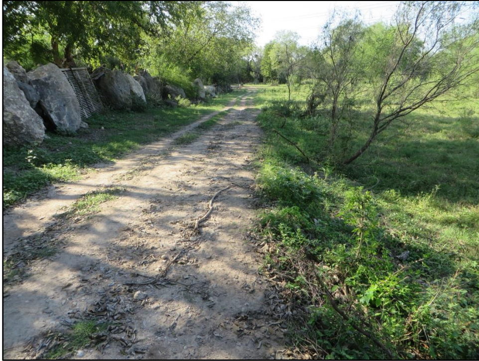
Figure 36. Two-track dirt road constructed on an earthen berm and bordered by bedrock boulders, facing south.
