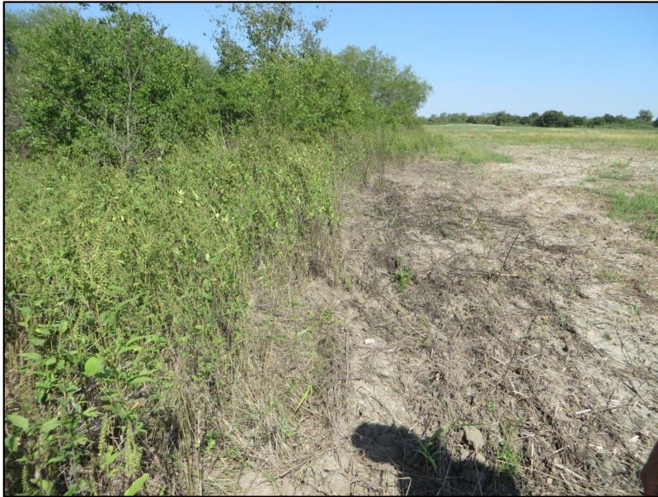
Figure 22. Overview of existing SAWS sewer easement along the northern APE segment, facing north.
