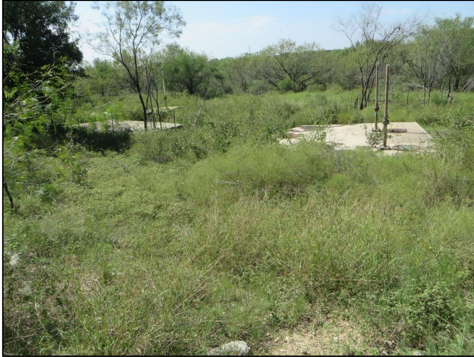
Figure 3. Existing pump station and tie-in location at southern APE terminus, facing west.
