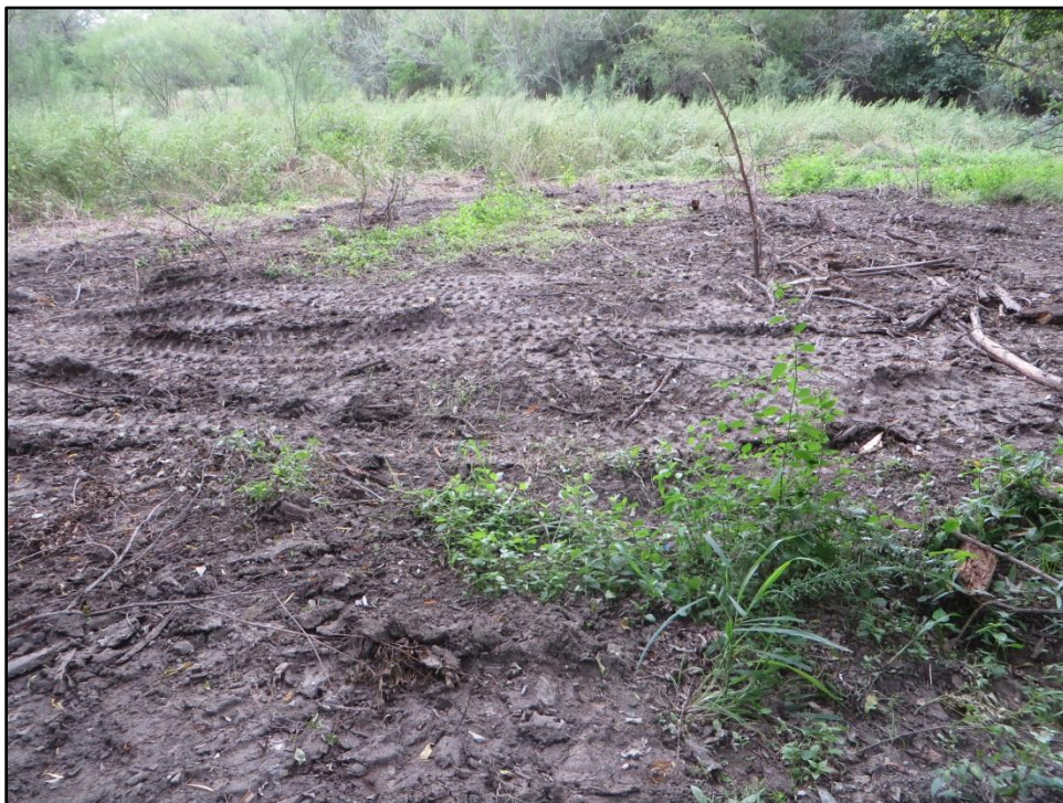
Figure 29. Vegetation clearing near AG23, facing southeast.
