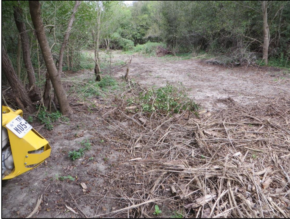
Figure 28. Vegetation clearing near AG22, facing northwest.
