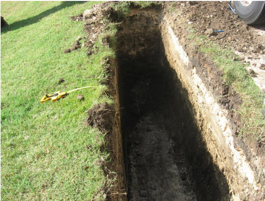
Photo #7: Facing west toward GT #3. Note the chalk bedrock in the bottom of the trench
