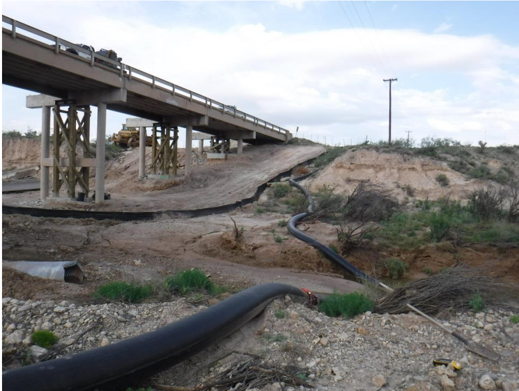
Figure 4-6. Active Construction at Salt Creek Crossing, Facing Southwest.
