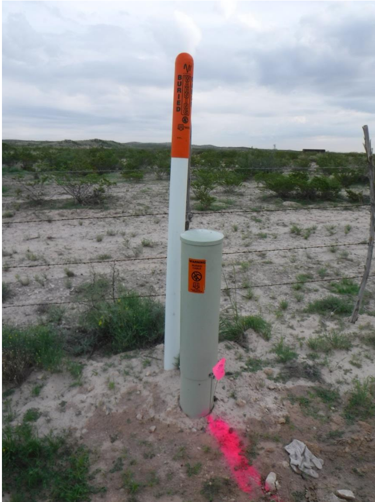
Figure 4-7. Buried Cable Warning at Eastern Side of Salt Creek Crossing, Facing North.
