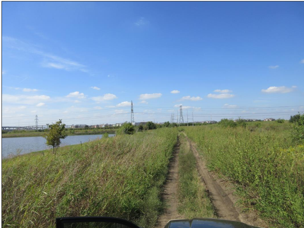
Figure 6: Overview of South launch and pond to the south; facing southeast.
