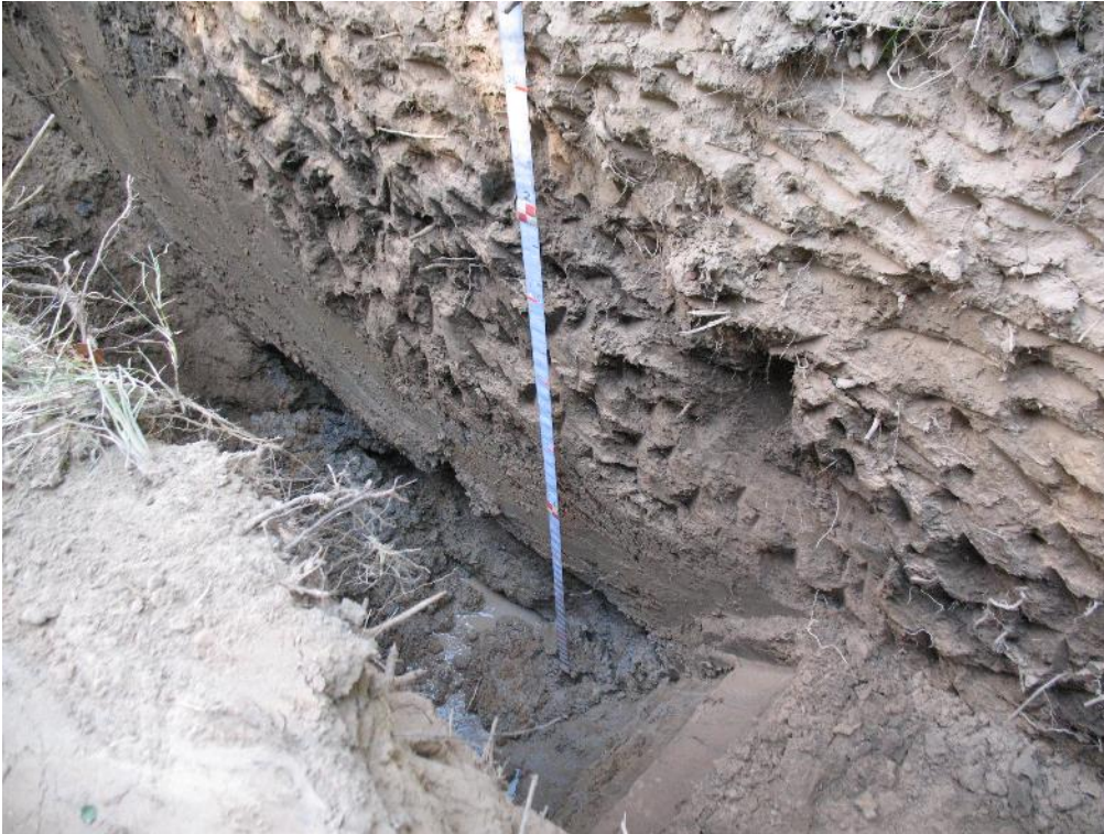
Figure 9. Soil profile of BHT 4. Note water table and slumping at bottom of trench.
