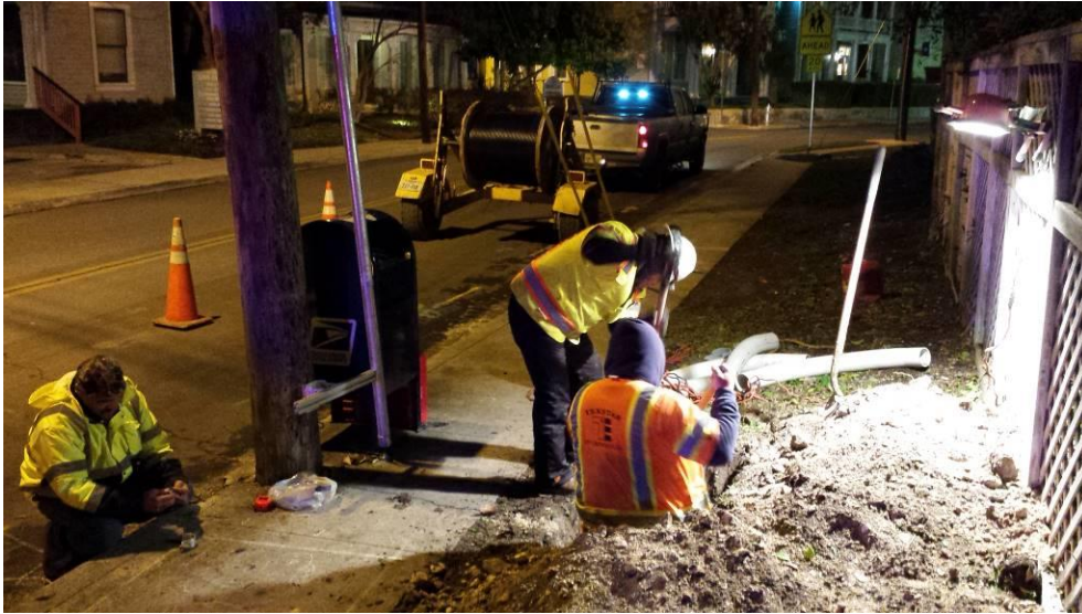
Photo #1: View north along South Presa with construction crew excavating Trench 1.
