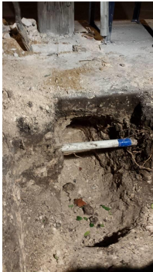
Photo #4: Westerly hand-excavated bore beneath sidewalk and irrigation line.
