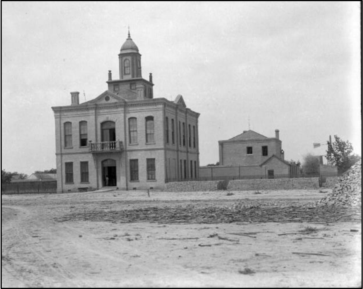
Figure 4-11. Old County Courthouse and Jail in a late nineteenth century photograph. Photo is facing north. Note the wall surrounding the Jail and guard house structure just in front of the Jail.
