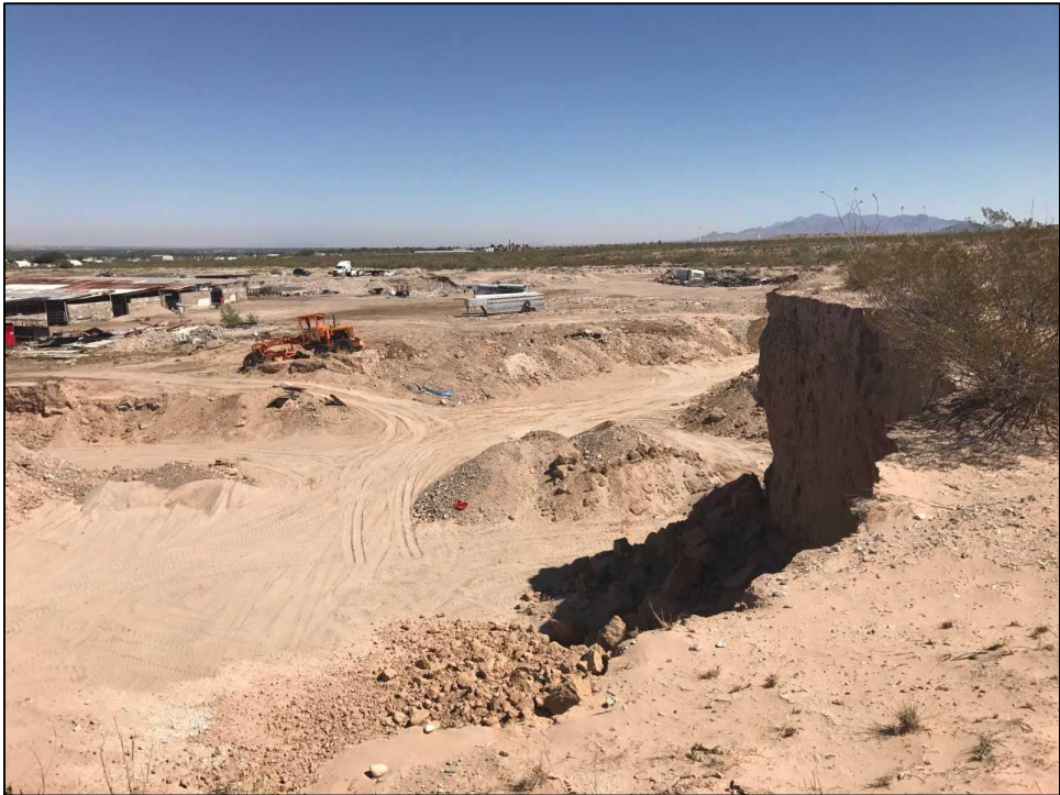
Figure 4-3. Project area impacted by construction looking north; note undercut slope at right.
