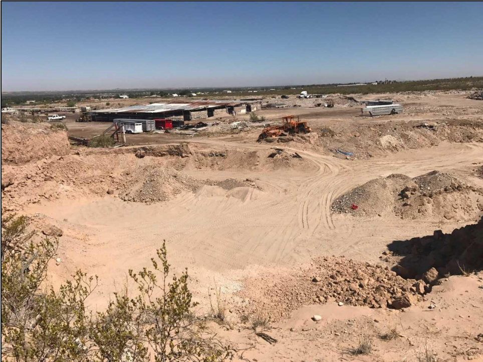
Figure 4-4. Project area impacted by construction looking north-northwest; note bulldozing/grading.
