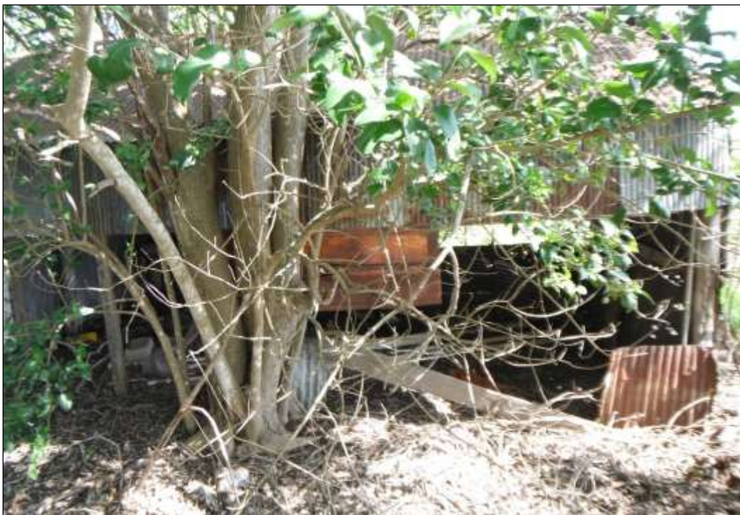
Figure 6-13. Structure W1-E (41HY536)—Front of Eastern Barn (Facing Northeast)
