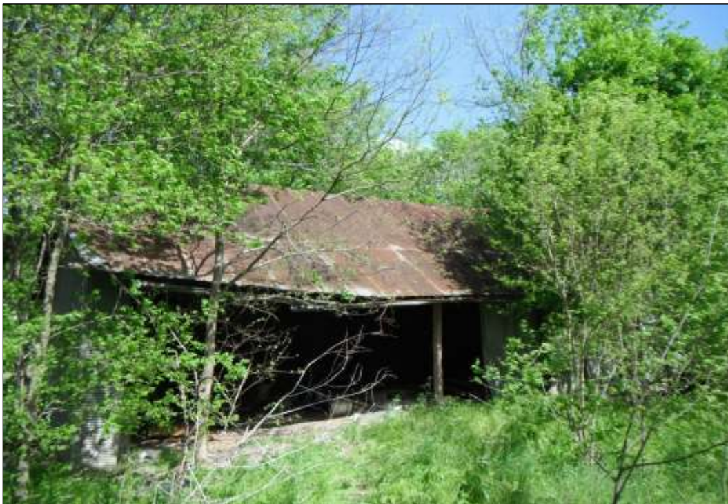
Figure 6-9. Structure W1-D (41HY536)—Front of Central Barn (Facing Northwest)
