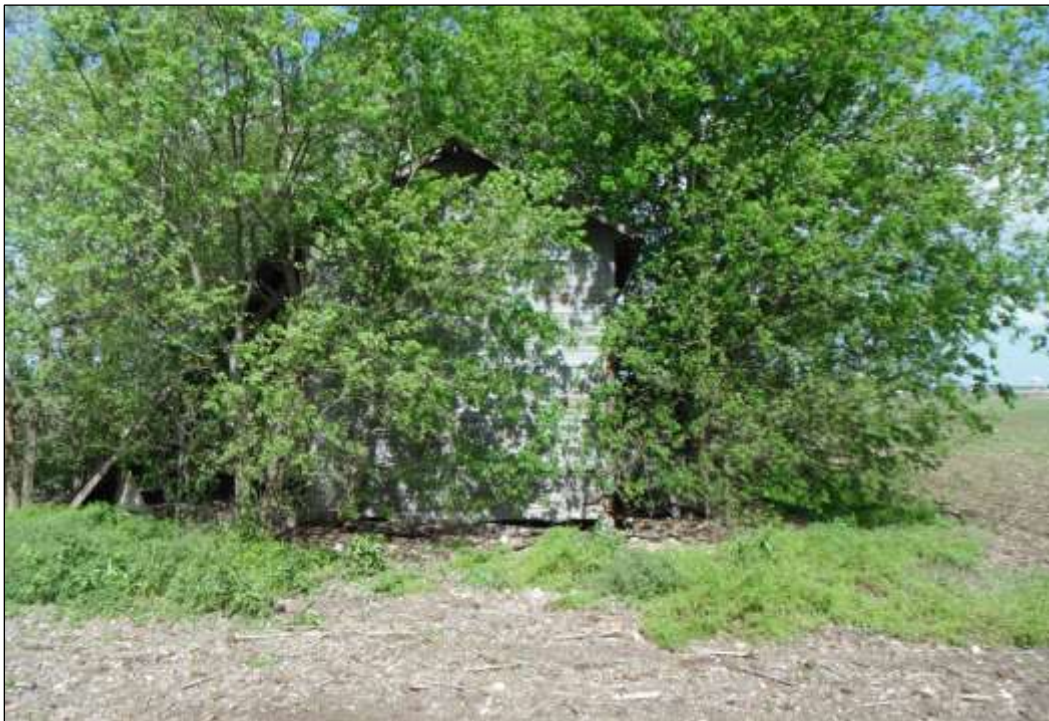
Figure 6-7. Structure W1-B (41HY536)—Side of Barn (Facing Southwest)
