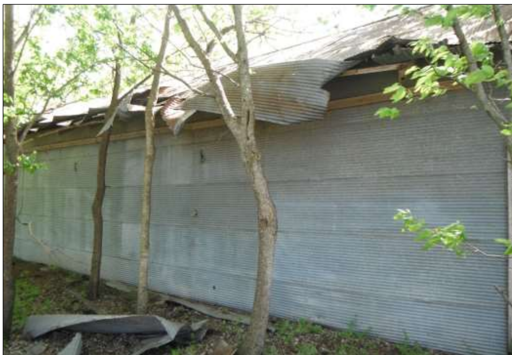
Figure 6-11. Structure W1-D (41HY536)—Back of Central Barn (Facing East)
