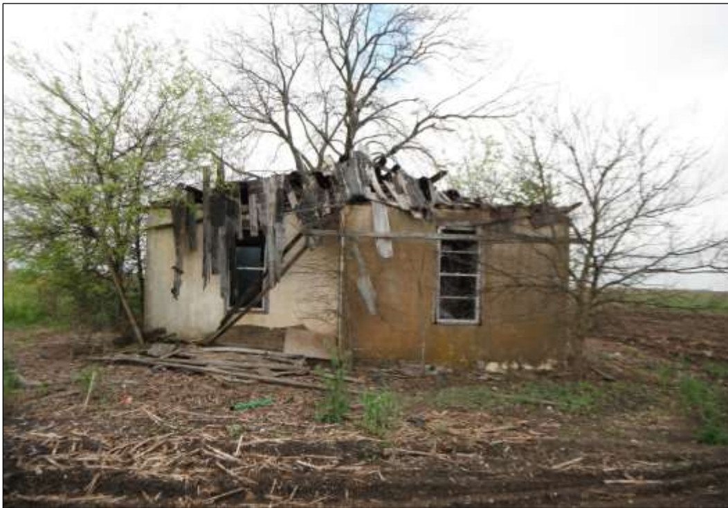
Figure 6-23. Structure W2 (41HY537)—Northeastern Side of House (Facing Southwest)
