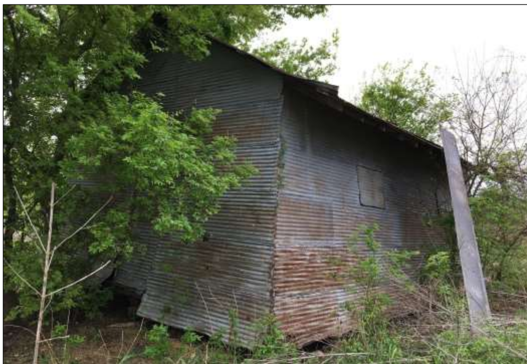
Figure 6-72. Structure W7 (41HY542)—Northeastern Corner of Barn (Facing Southeast)
