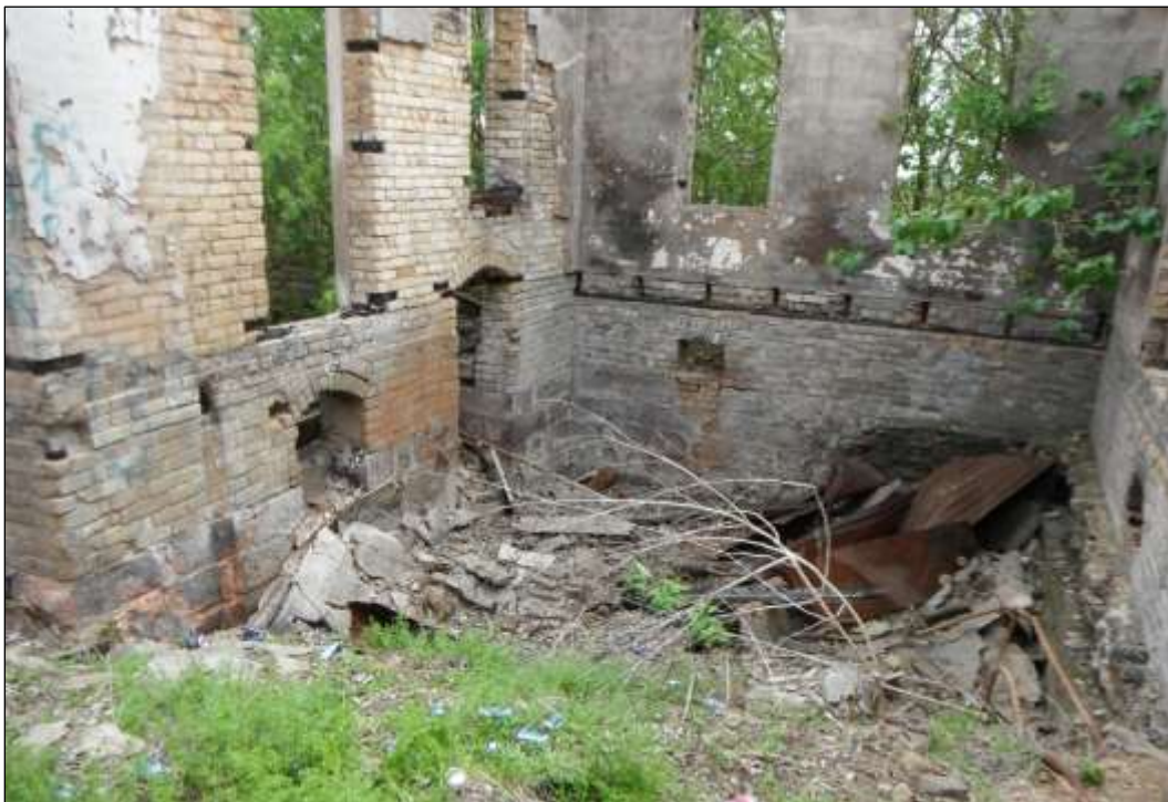
Figure 6-62. Structure W6-A (41HY541)—Southeastern Room and Basement Interior (Facing Southeast)
