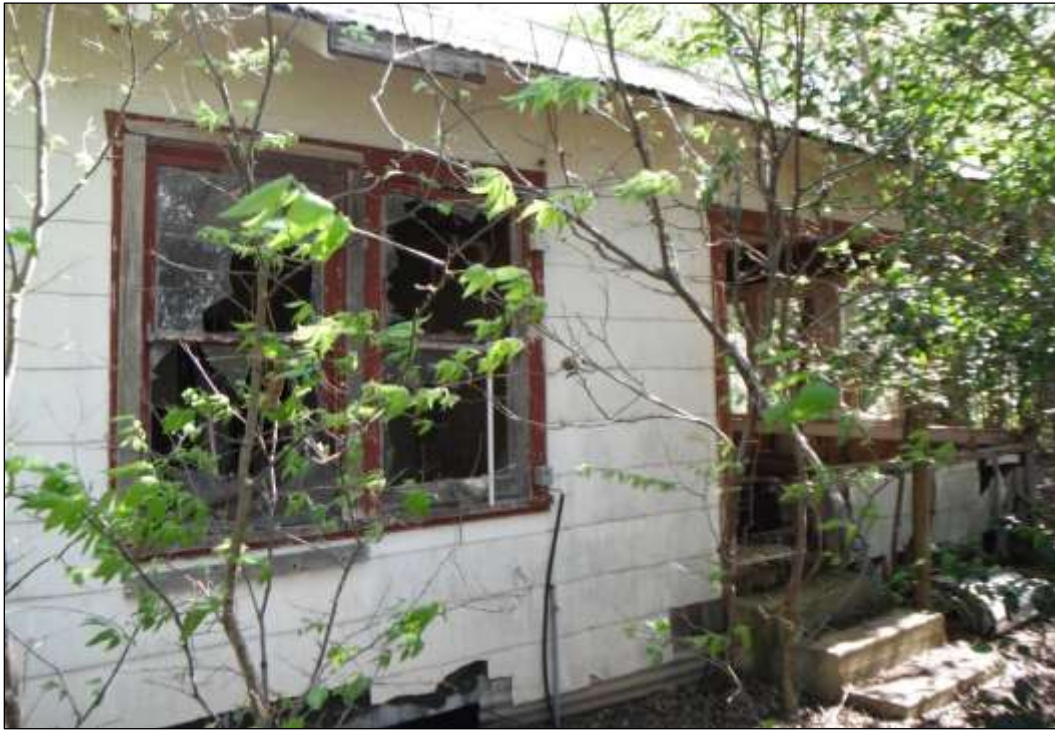
Figure 6-4. Structure W1-A (41HY536)—Side of House (Facing Northeast)
