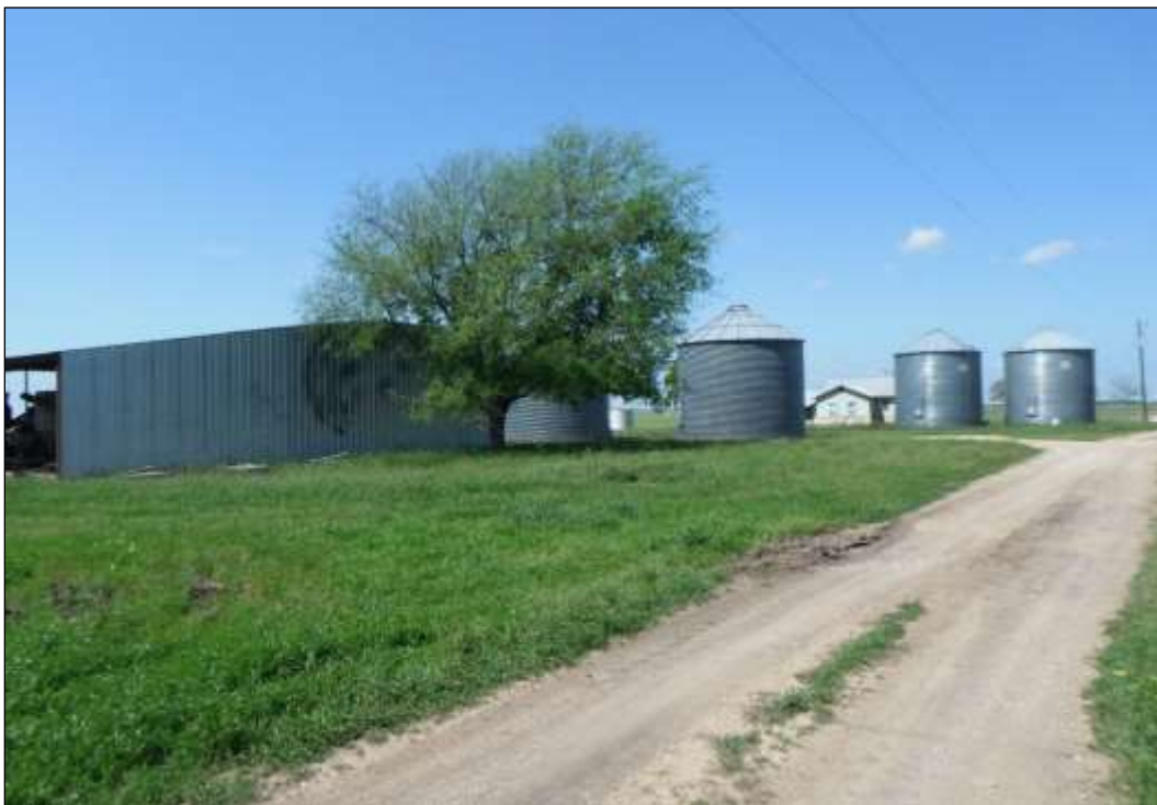
Figure 6-46. Modern Equipment Barn and Storage Silos on Site 41HY539 (Facing South)
