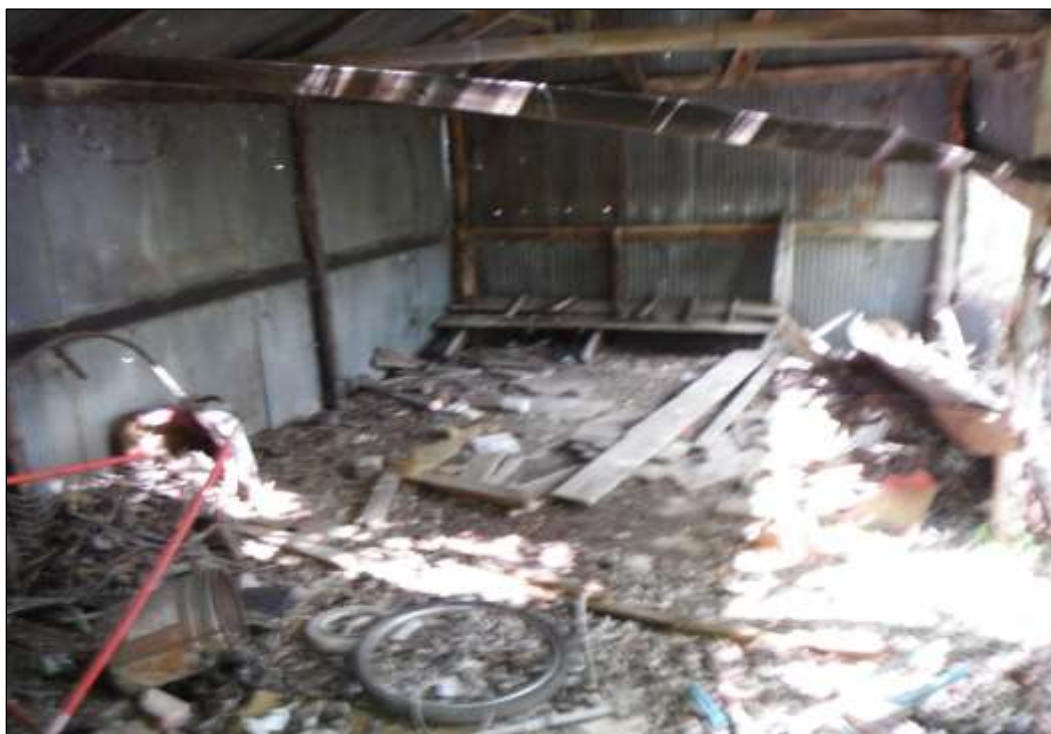
Figure 6-17. Structure W1-F (41HY536)—Interior of Northeastern Barn (Facing Northeast)
