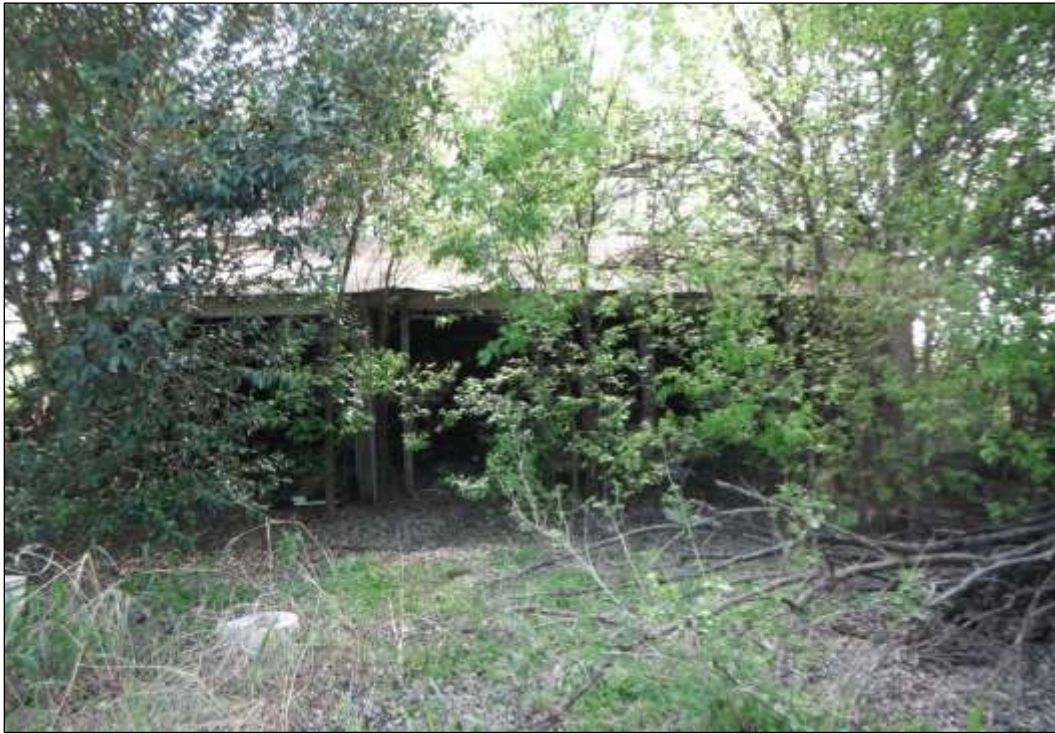
Figure 6-67. Structure W6-C (41HY541)—Front of Barn (Facing Southwest)
