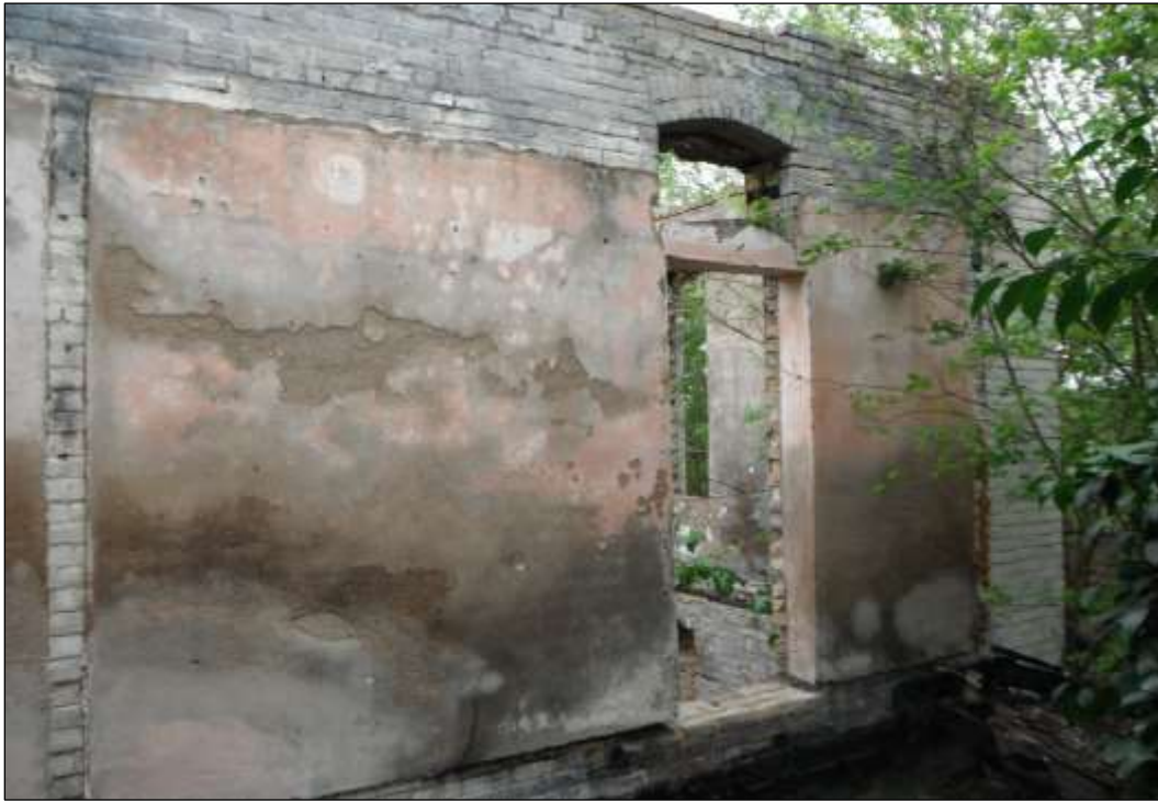
Figure 6-59. Structure W6-A (41HY541)—East Half of South Side of House (Facing East)
