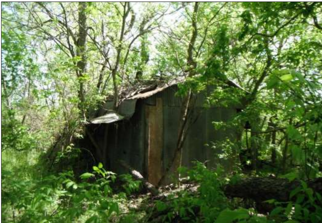
Figure 6-16. Structure W1-F (41HY536)—Corner of Northeastern Barn (Facing Northeast)
