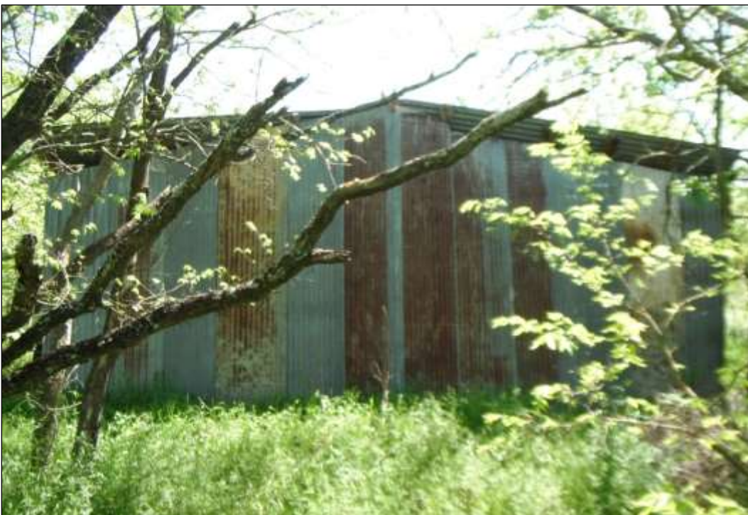
Figure 6-43. Structure W4-C (41HY539)—Northwestern Side of Barn (Facing Southeast)
