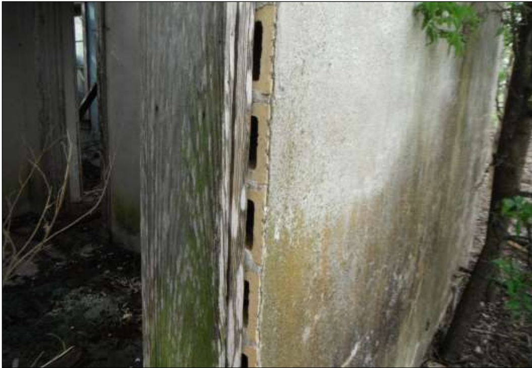
Figure 6-25. Structure W2 (41HY537)—Detail of Clay Tile Construction
