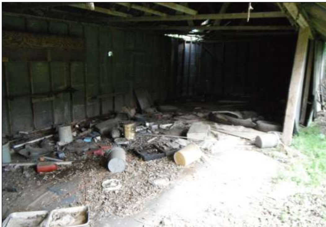
Figure 6-10. Structure W1-D (41HY536)—Interior of Central Barn (Facing North)
