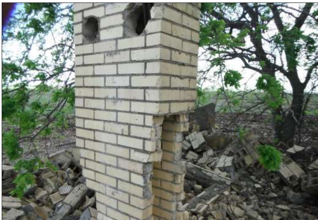
Figure 6-51. Detail of Chimney Base on Site 41HY540 (Facing South)
