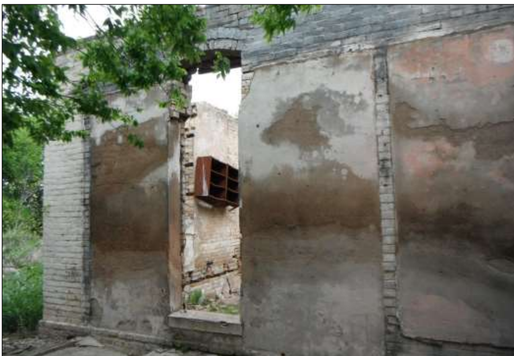
Figure 6-58. Structure W6-A (41HY541)—West Half of South Side of House (Facing North)
