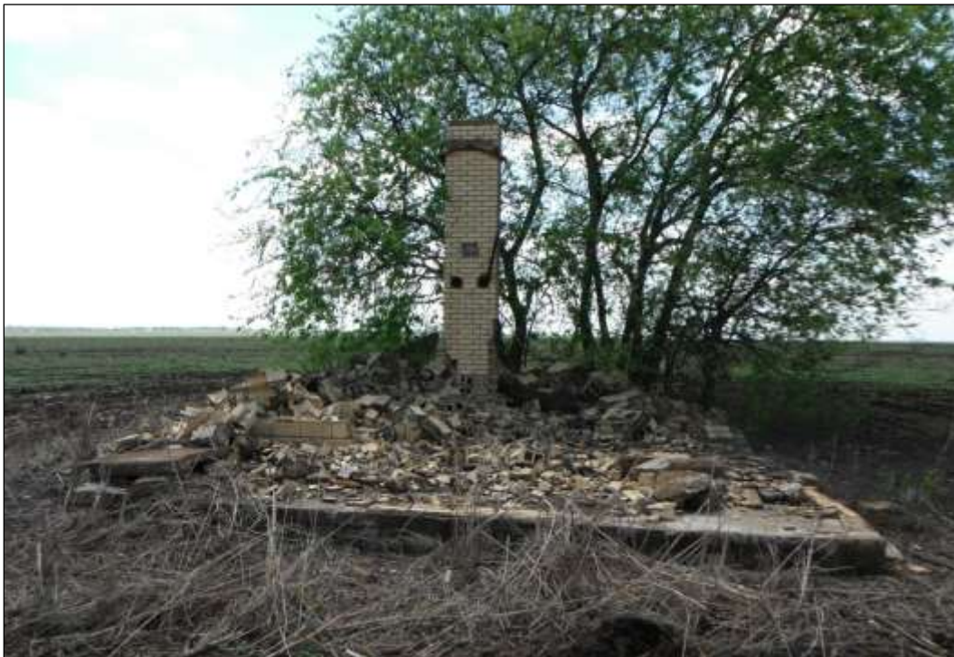
Figure 6-49. House Foundation and Chimney on Site 41HY540 (Facing Southwest)
