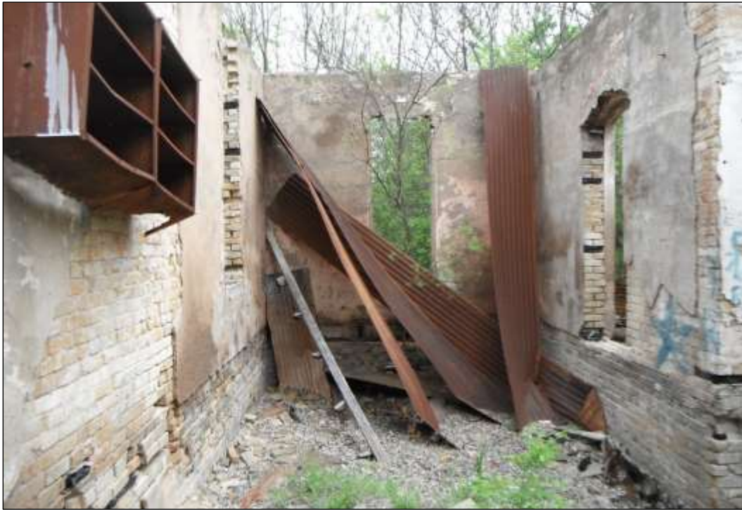
Figure 6-61. Structure W6-A (41HY541)—Northeastern Room Interior (Facing Northeast)
