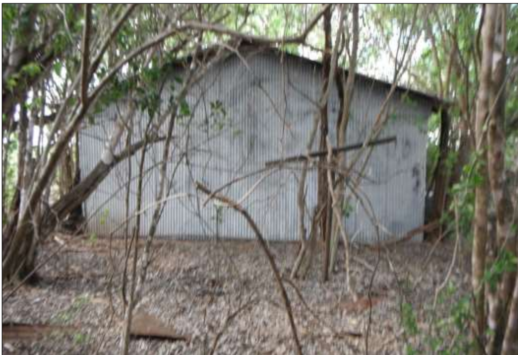
Figure 6-68. Structure W6-C (41HY541)—Southeastern End of Barn (Facing Northwest)
