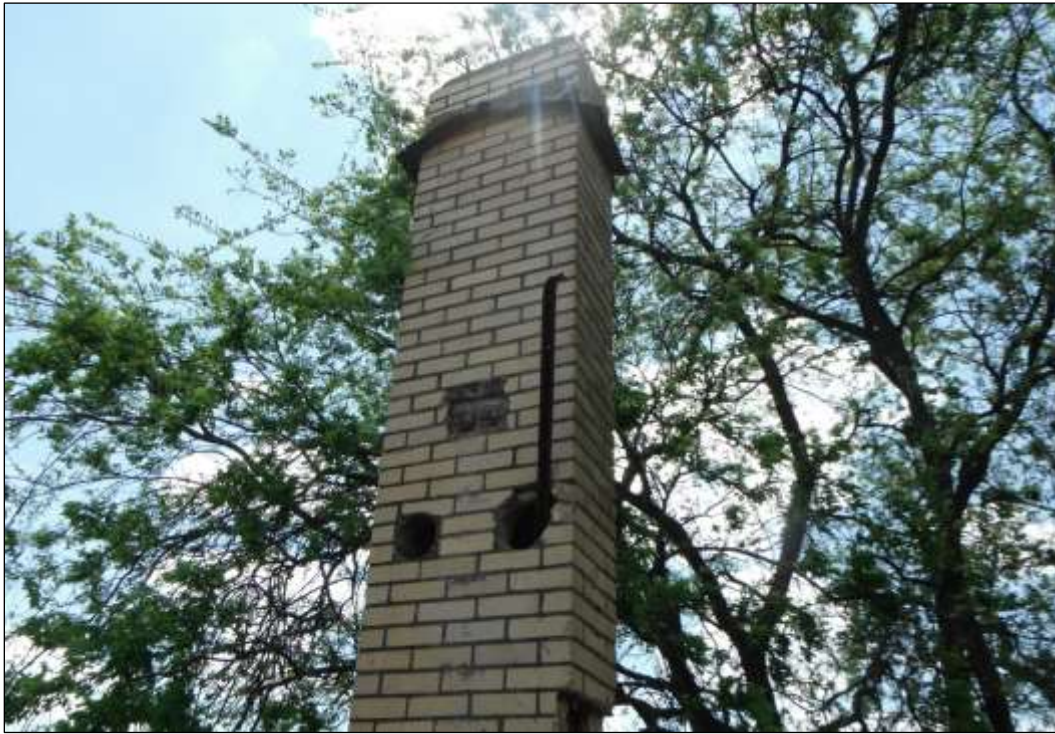
Figure 6-52. Detail of Chimney Top on Site 41HY540 (Facing South)
