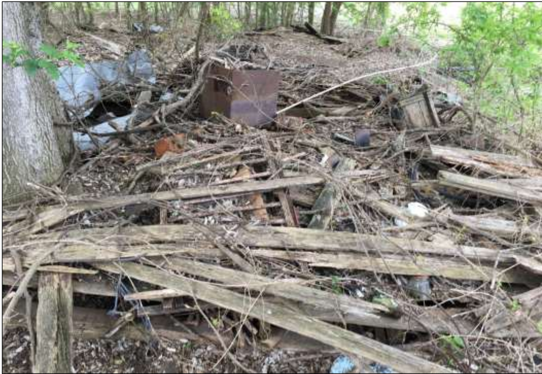
Figure 6-73. Collapsed Structure on Site 41HY542 (Facing Southwest)
