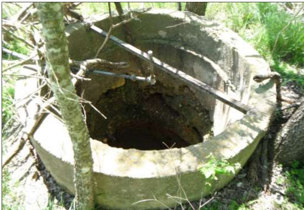
Figure 6-44. Concrete Well near Structure W4-C on Site 41HY539 (Facing West)
