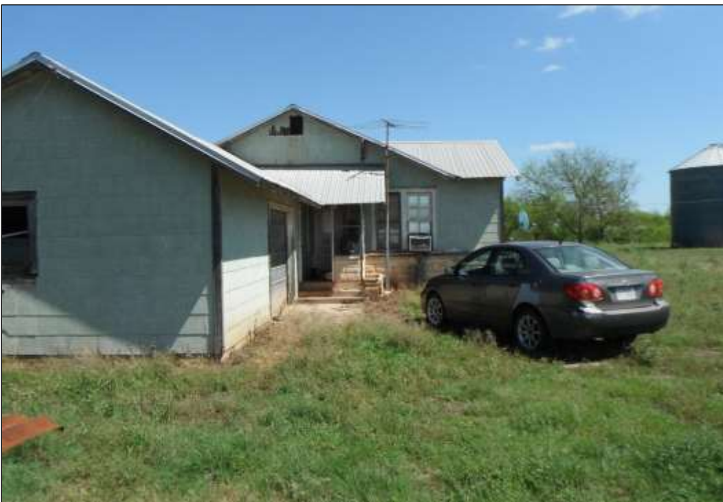
Figure 6-39. Structure W4-A (41HY539)—Back of House (Facing Northeast)
