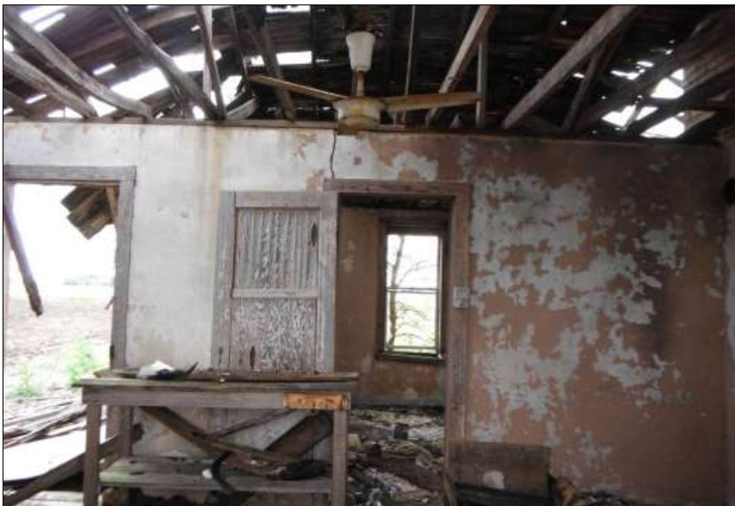
Figure 6-24. Structure W2 (41HY537)—Interior of House (Facing Northeast)
