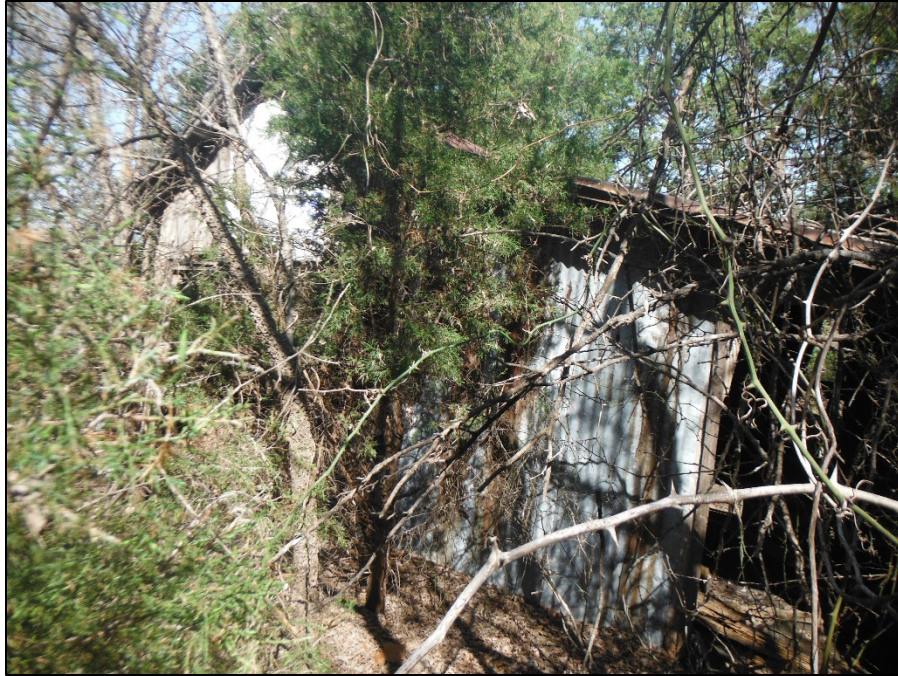
Figure 11. View of south wall of Feature 1 at site 41COL270. View to northwest.
