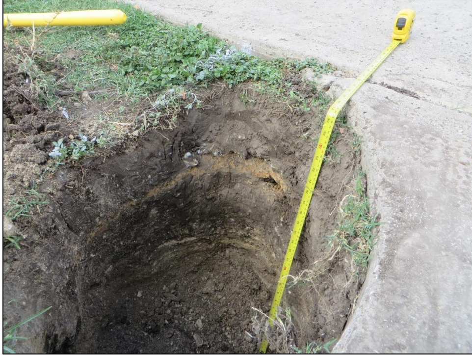
Figure 10. North wall profile of BP2; facing north.
