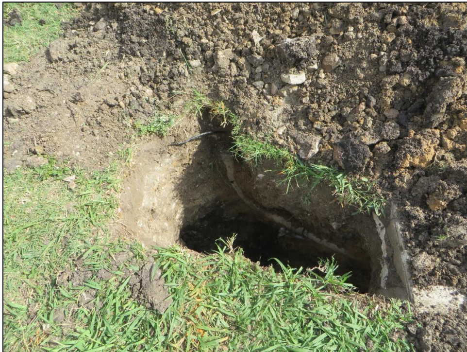
Figure 11. Overview of BP 2, showing pipe within the profile; facing east.
