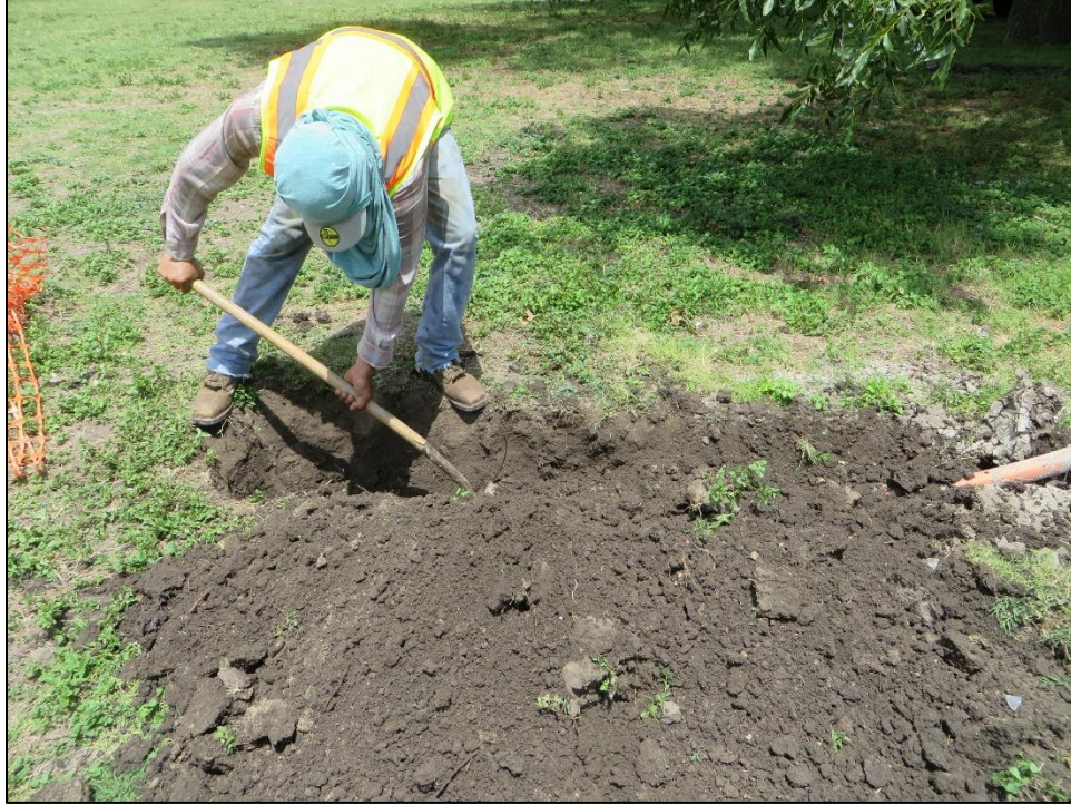
Figure 13. Overview of the excavation of BP 4; facing north.
