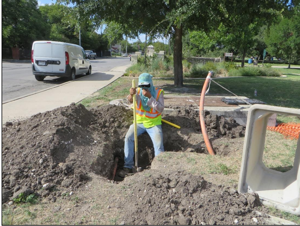
Figure 6. Excavation of the handhole; facing north.
