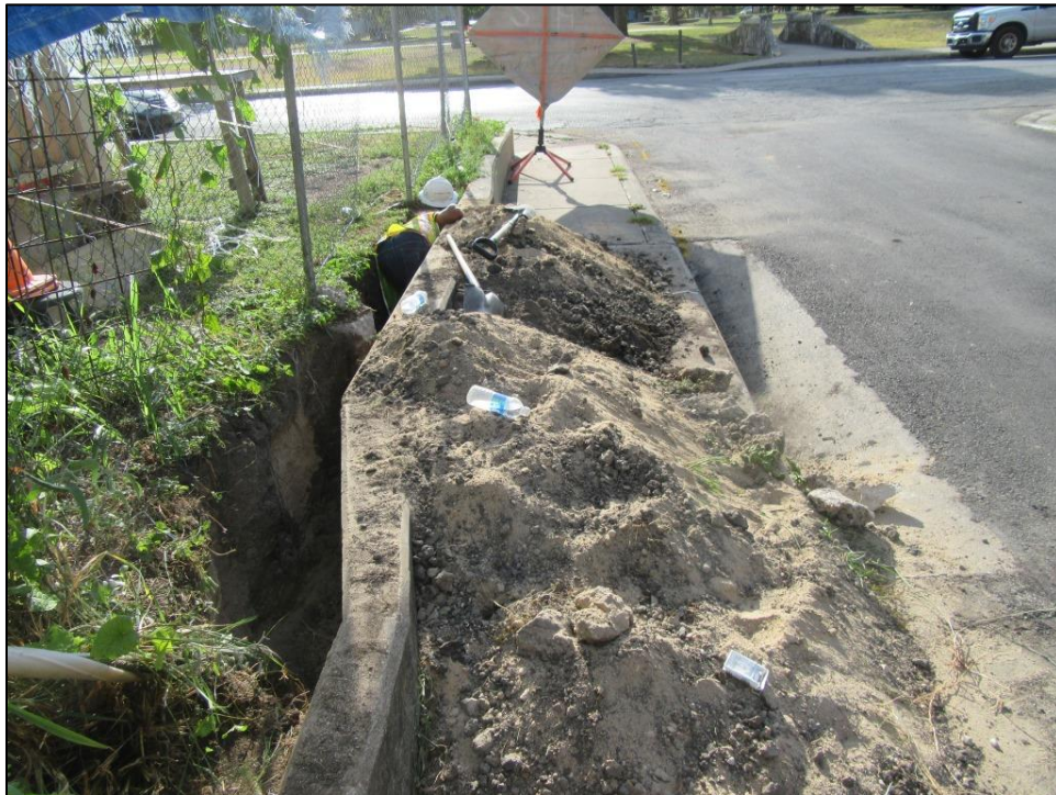
Figure 8. View soils from trench along Kempkau.
