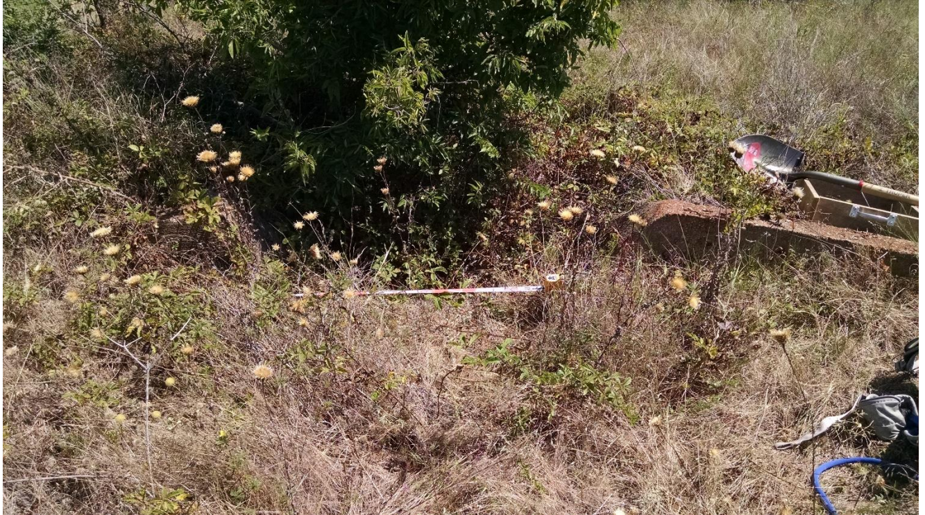
Photo 10. Isolated concrete agricultural drainage feature, looking downslope. View to the north.
