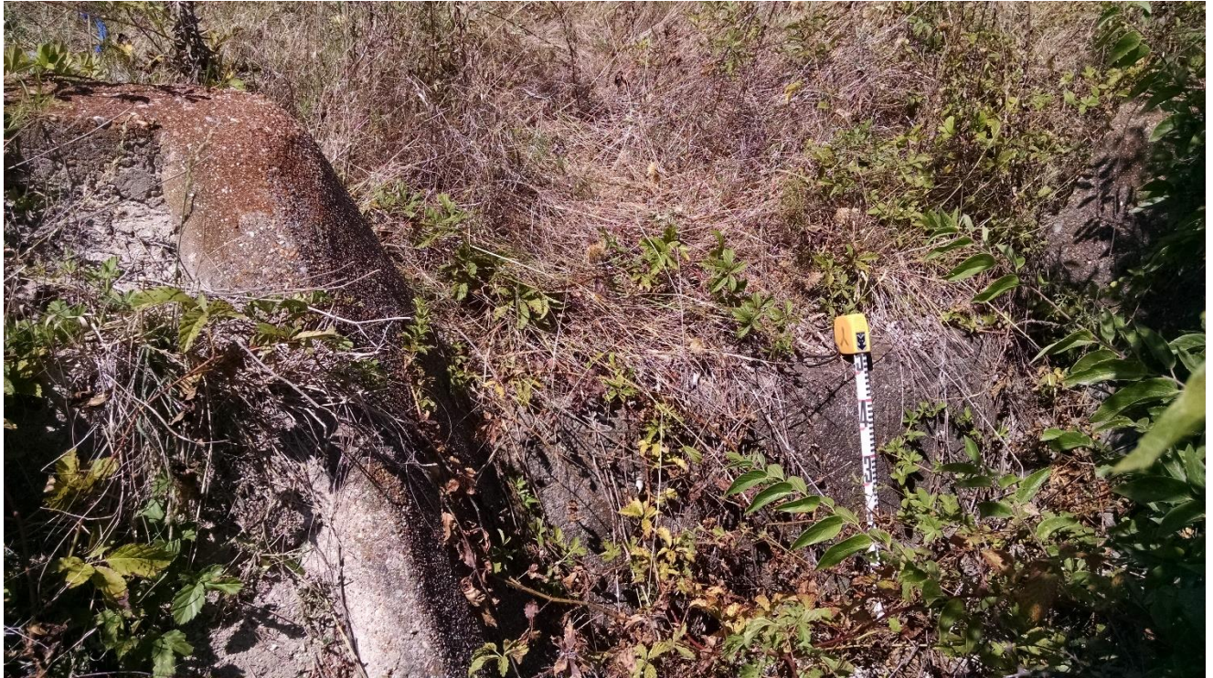
Photo 9. Isolated concrete agricultural drainage feature, looking upslope. View to the south.
