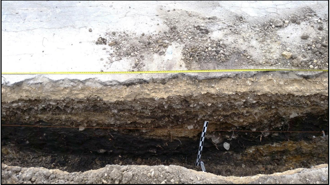
Figure 5-4. North wall profile of the SAWS trench with the Acequia de Valero .
