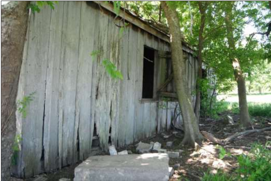
Figure 6-45. Resource 2—View of Northern (Rear) Façade of House (Facing Southwest)
