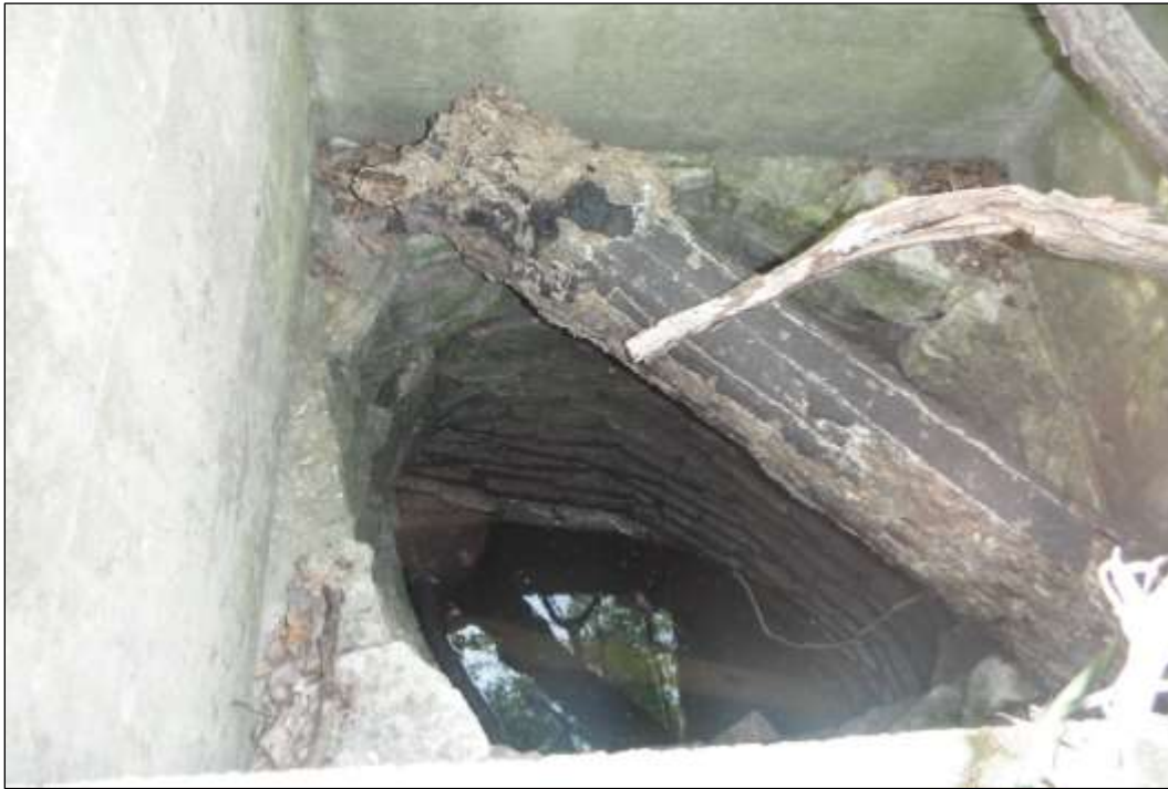
Figure 6-65. Interior of Limestone Well (Facing East)
