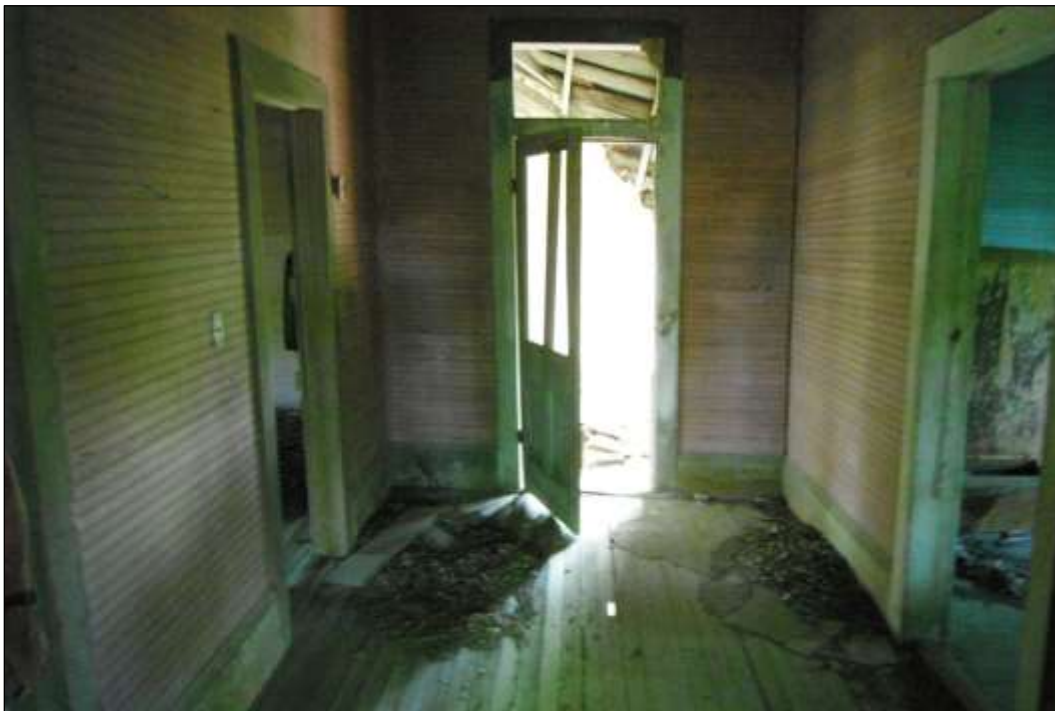
Figure 6-13. View of the Exterior Breezeway Door ( note transom ) (Facing West)
