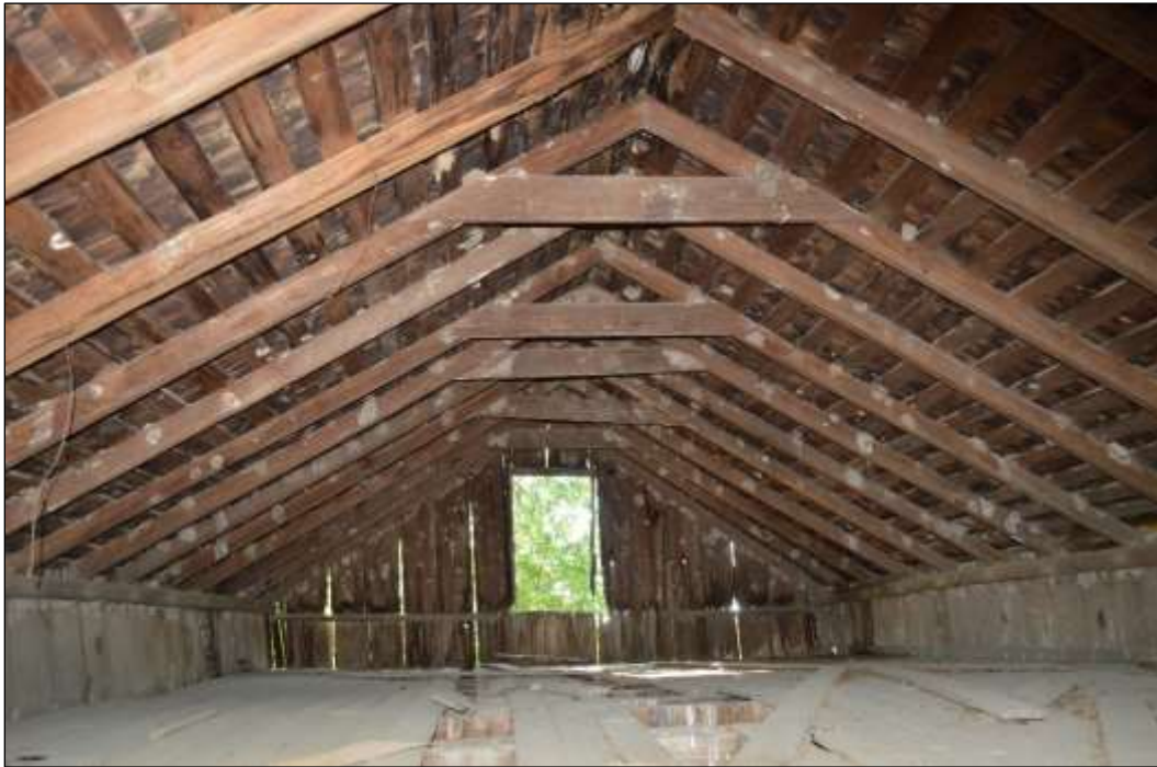
Figure 6-51. Resource 2—View of Second-Story Sleeping Loft (Facing East)
