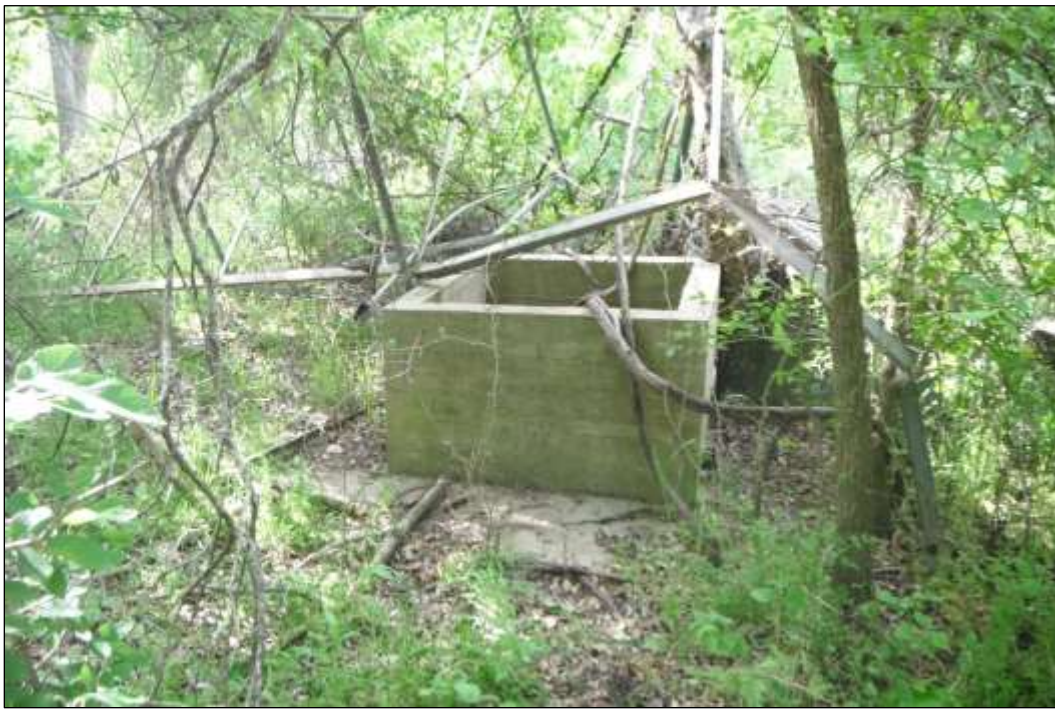
Figure 6-64. View of Limestone Well on Site 41TV2519 (Note Collapsed Windmill on Top) (Facing South)
