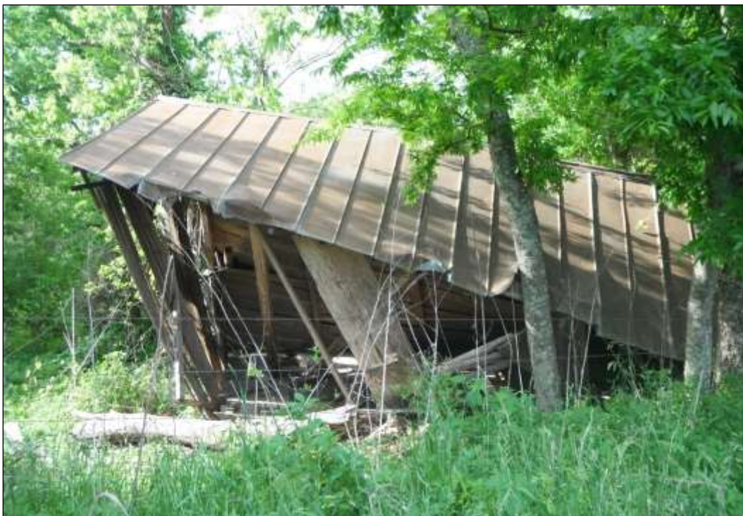
Figure 6-63. Resource 3B—View of the Barn (Facing South)
