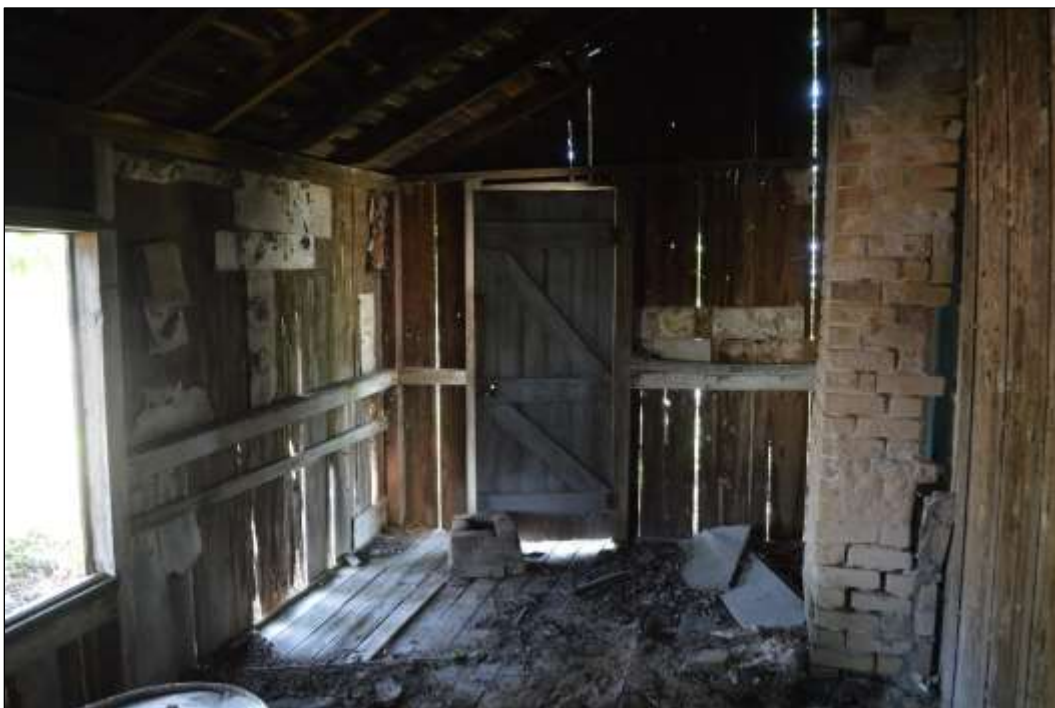
Figure 6-53. Resource 2—View of Northeastern Room (Note Flue at Right) (Facing East)
