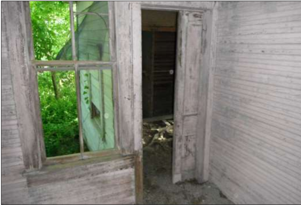
Figure 6-17. Resource 1A—Door Leading from Mater Bedroom to Child's Bedroom (Facing North-Northeast)
