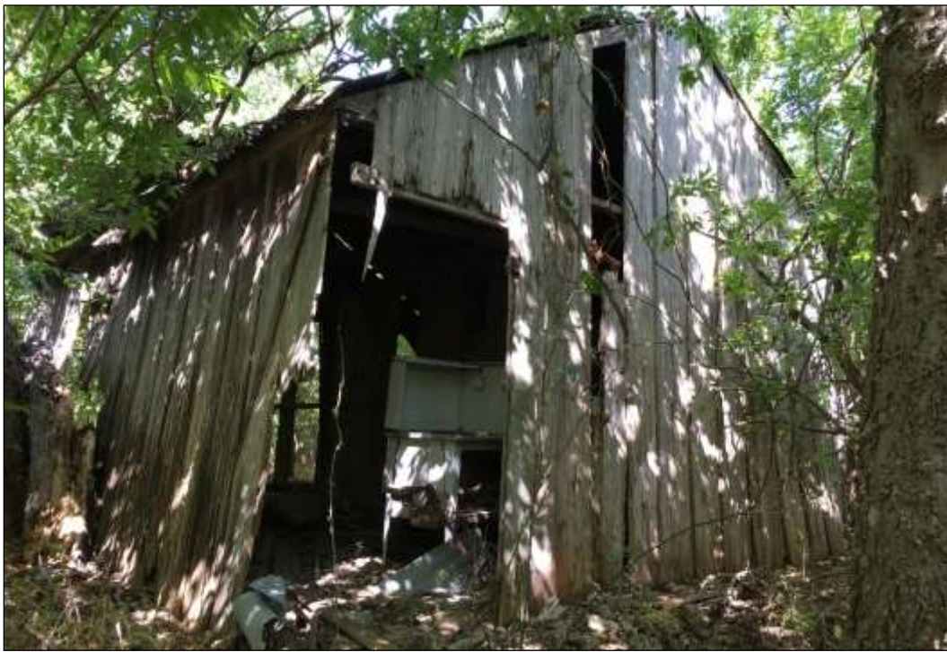
Figure 6-76. Resource 4—View of Rear Façade of Garage (Facing West)
