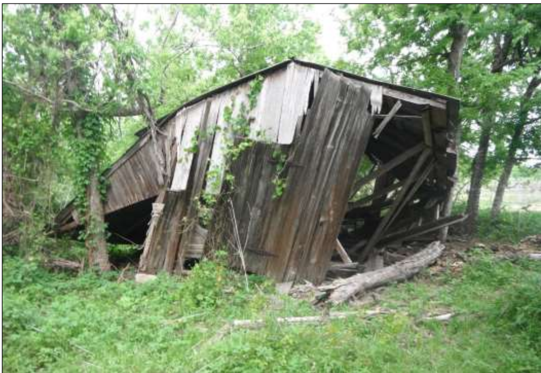
Figure 6-61. Resource 3B—View of the Barn (Facing West)
