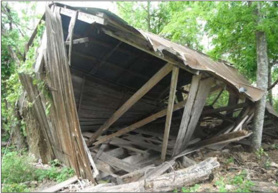
Figure 6-62. Resource 3B—View of the Barn (Facing Southwest)
