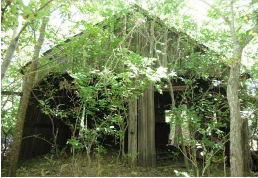
Figure 6-75. Resource 4—View of Front Façade of Garage (Facing Northeast)
