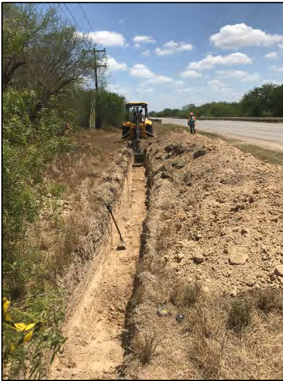
Figure 15. BHT 1 on 41MC372, facing west.
