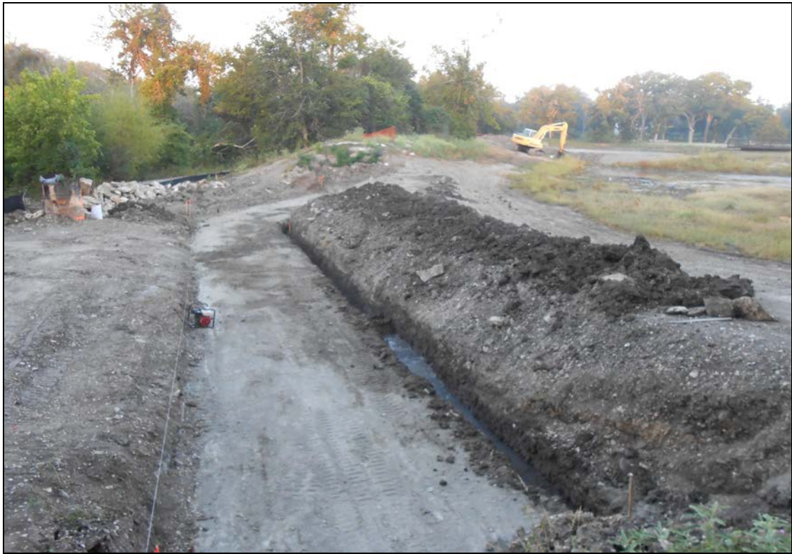
Figure 7. View of soil barrier and trench for new concrete dam.
