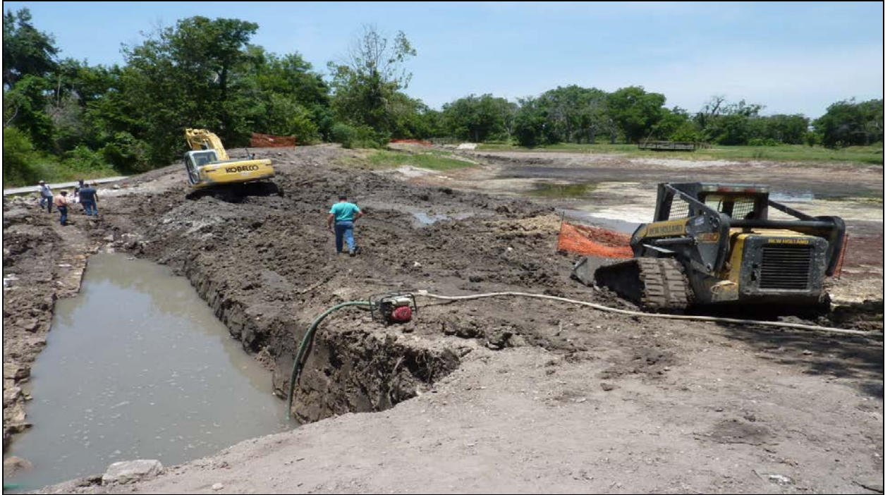
Figure 4. View of the old dam wall on the left side of the water, new trench upslope from the historic dam wall.
