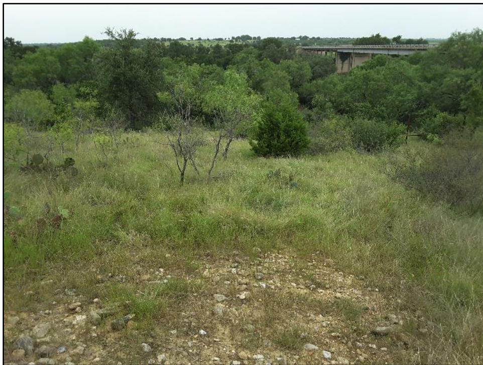
Figure 17. Overview of 41MI2 with FM 45 bridge at the Colorado River, facing south.
