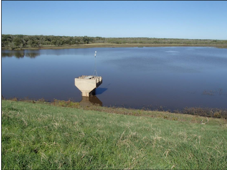
Figure 26. Inlet at FRS 21. Facing north.
