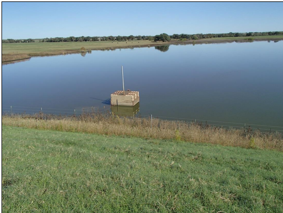
Figure 36. Inlet at FRS 28. Facing northeast.
