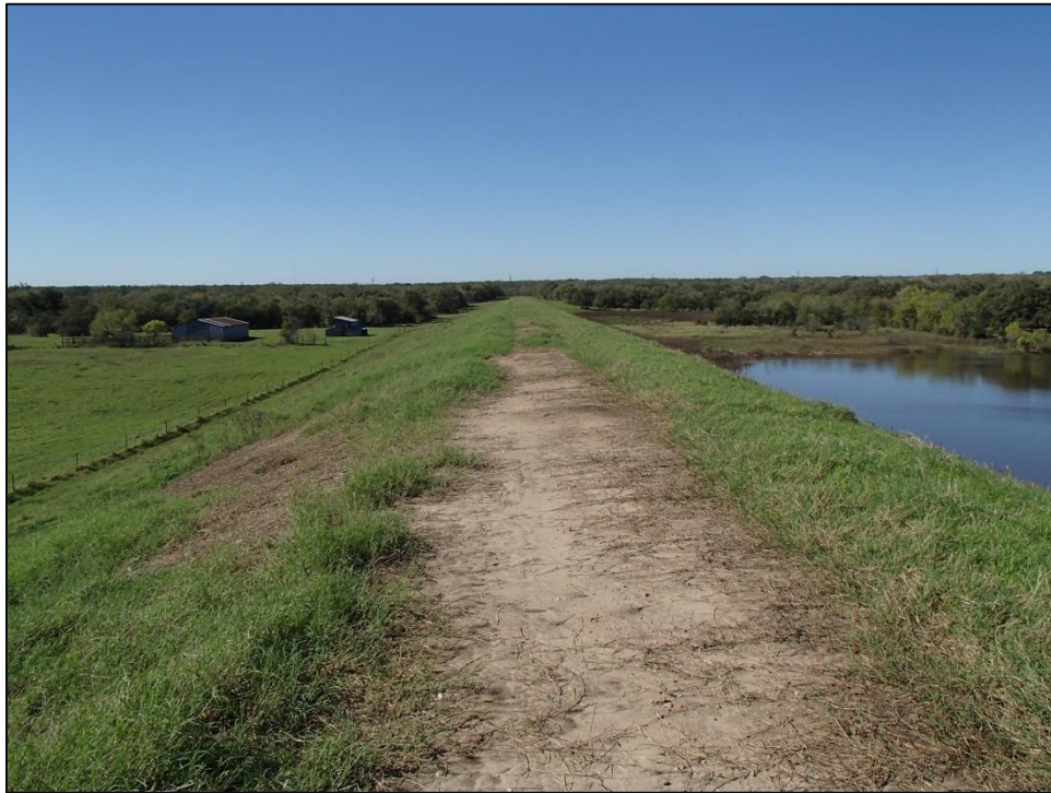
Figure 25. Earthen dam at FRS 21. Facing southwest.
