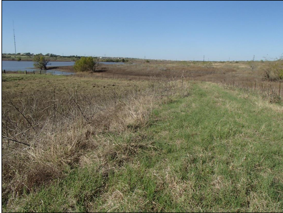
Figure 13. North end of auxiliary spillway. Facing north.
