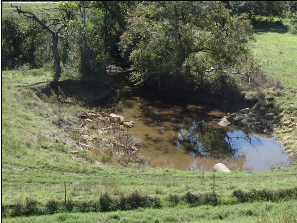
Figure 28. View of outlet pipe and plunge basin below dam. Facing south.
