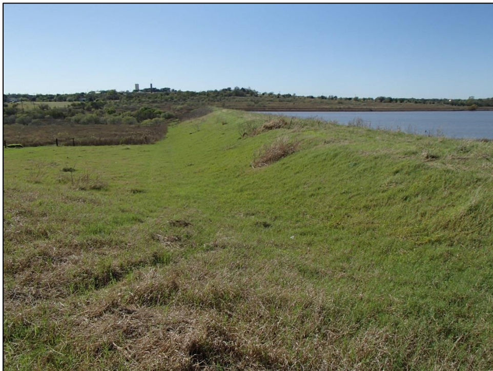
Figure 14. Earthen dam structure (FRS 10). Facing southwest.
