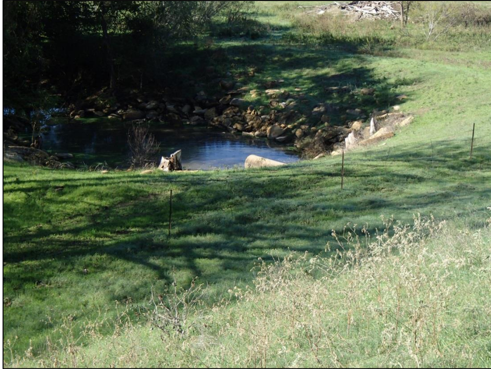
Figure 37. View of outlet pipe and plunge basin below dam. Facing southwest.
