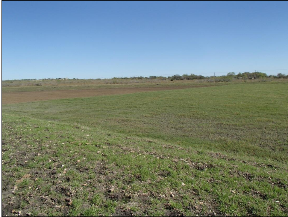
Figure 19. Overview of auxiliary spillway depression. Facing north.
