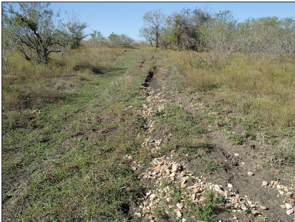
Figure 22. View of eroded and gullied access road leading up to dam where two artifacts were identified. Facing northwest.
