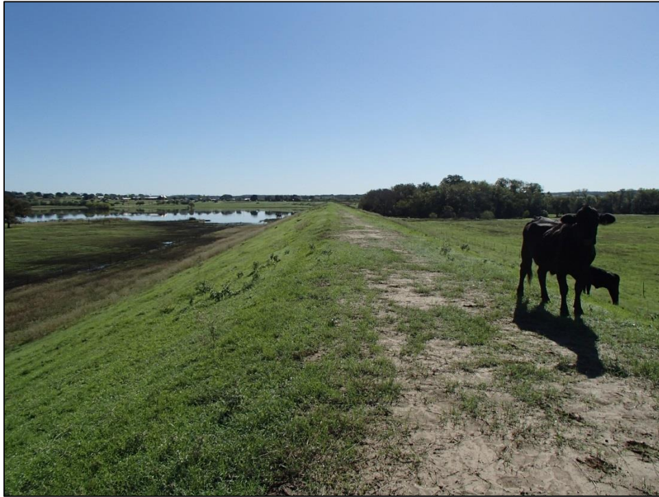
Figure 35. Earthen dam at FRS 28. Facing southeast.
