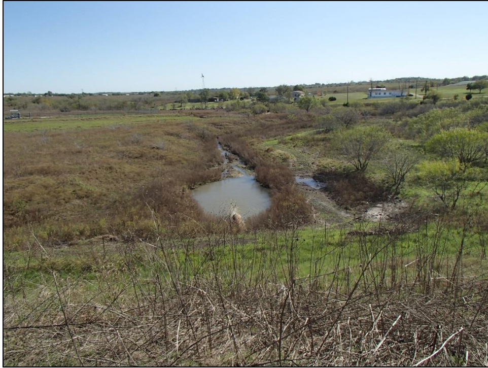
Figure 11. View of outlet pipe and plunge basin below dam. Facing south.
