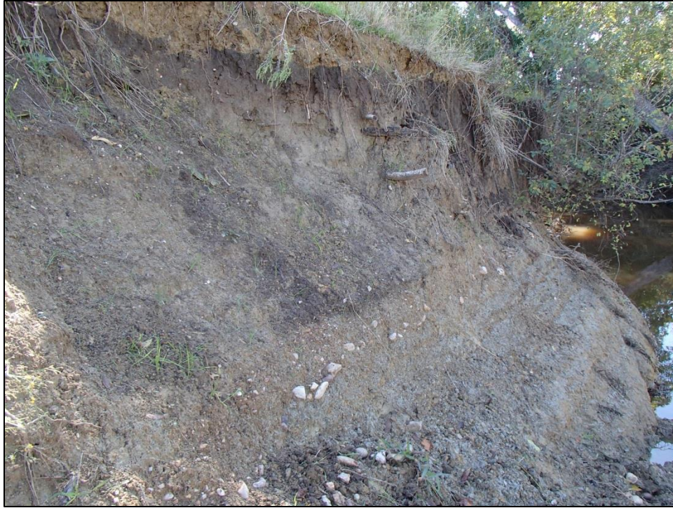
Figure 29. Cutbank exposure along channel below dam outlet. Facing south.
