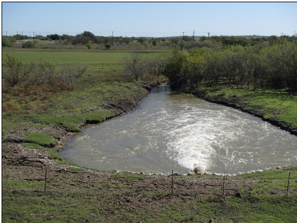
Figure 20. View of outlet pipe and plunge basin below dam. Facing southeast.
