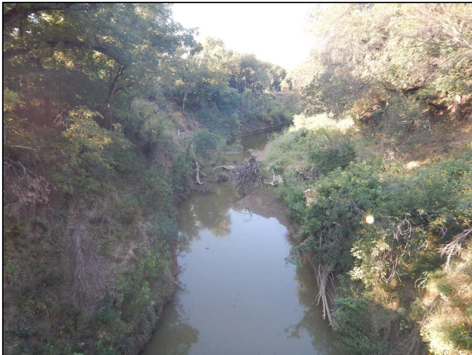
Figure 7. Overview Palo Pinto Creek upstream from bridge; facing southwest.
