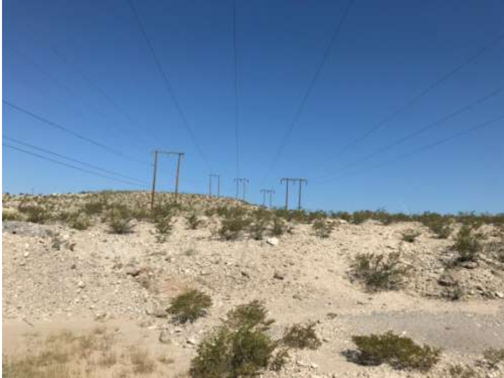
Figure 8. Overview of northern survey segment located just west of I10.
