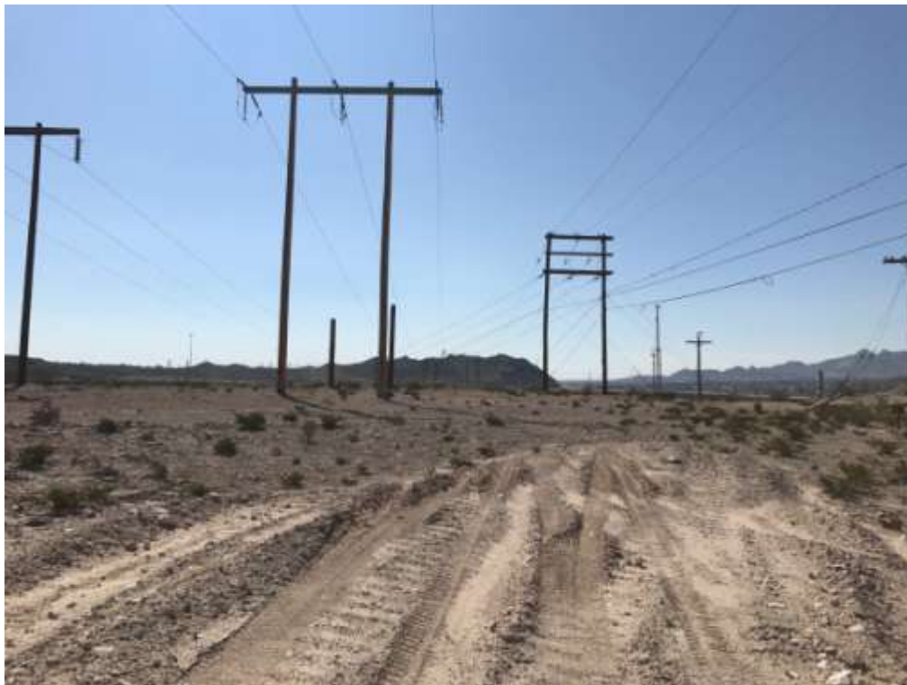
Figure 9. Overview of northern survey segment located just west of I10.
