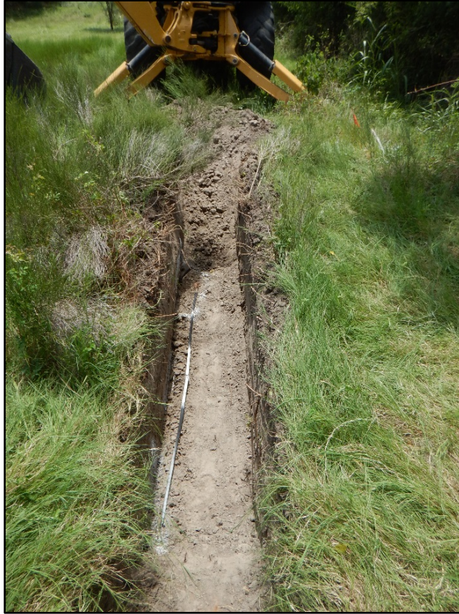
Figure 10. Overview of abandoned telephone line encountered in BHT02.
