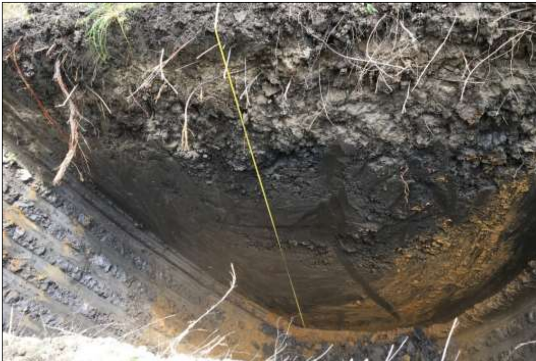
Figure A-2. Overview of Trackhoe Trench 2 (BHT-2)
