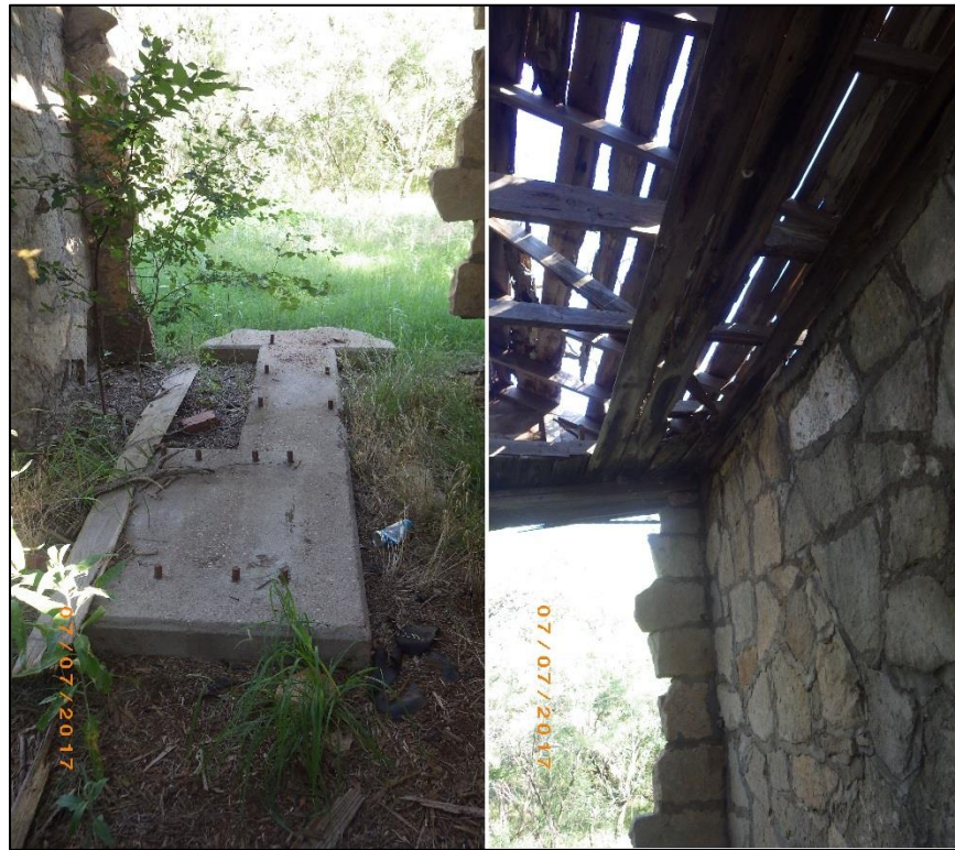
Figure 35. Interior of the small motor structure.
