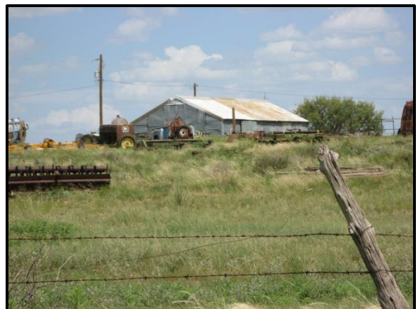
Barn on Farm Adjacent to the Project APE.
