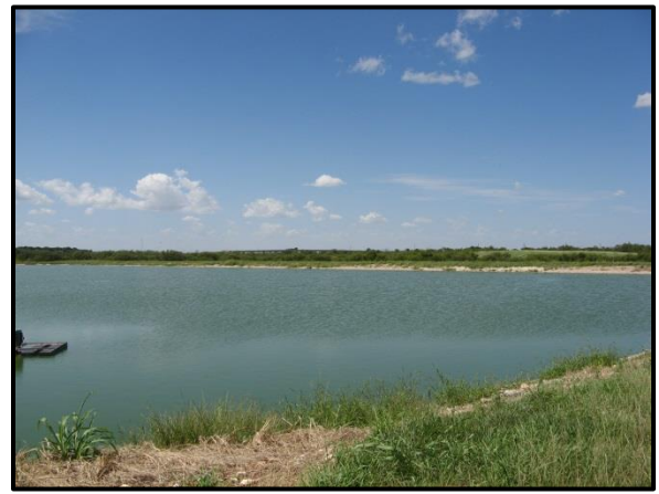
Exhibit 1. One of the Current WWTP Retention Ponds
