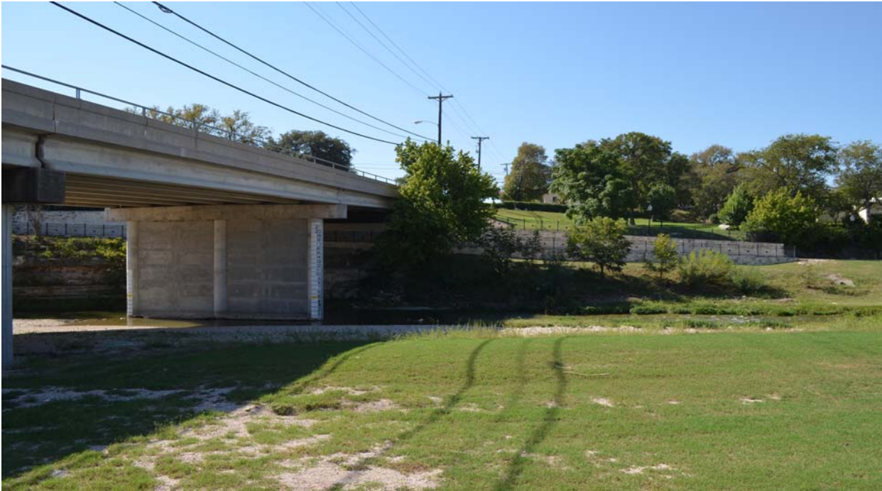
Figure 7. South view of Tract 1.
