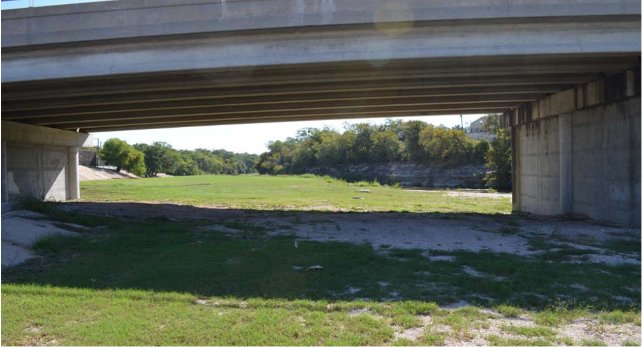
Figure 6. Eastern view of Tract 1 from bridge crossing. Note extensive gravel deposits.
