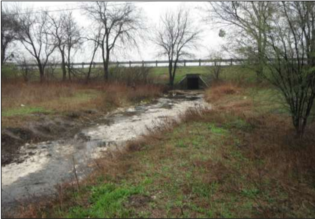
Figure 7. Unnamed Drainage Emerging from Culvert under FM 1825 (Facing South)
