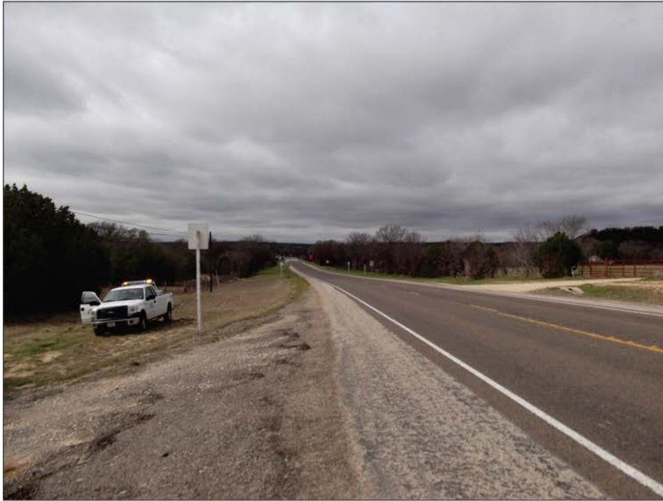
Figure 7. Looking south towards Cowhouse Creek. Note elevated section and drainage ditch.
