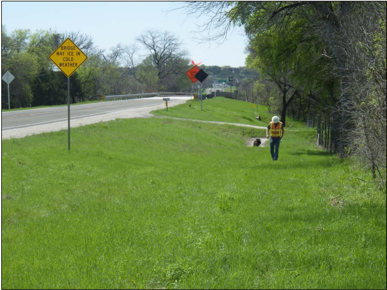
Figure 11: View looking south toward the bridge from the approximate location of BT4, showing ditching and wide fill section of the ROW in proximity to the bridge.
